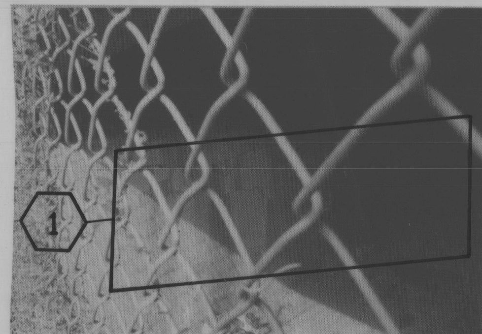
PHOTO N°2 ABUTMENT N°1 Southend - Eastside
