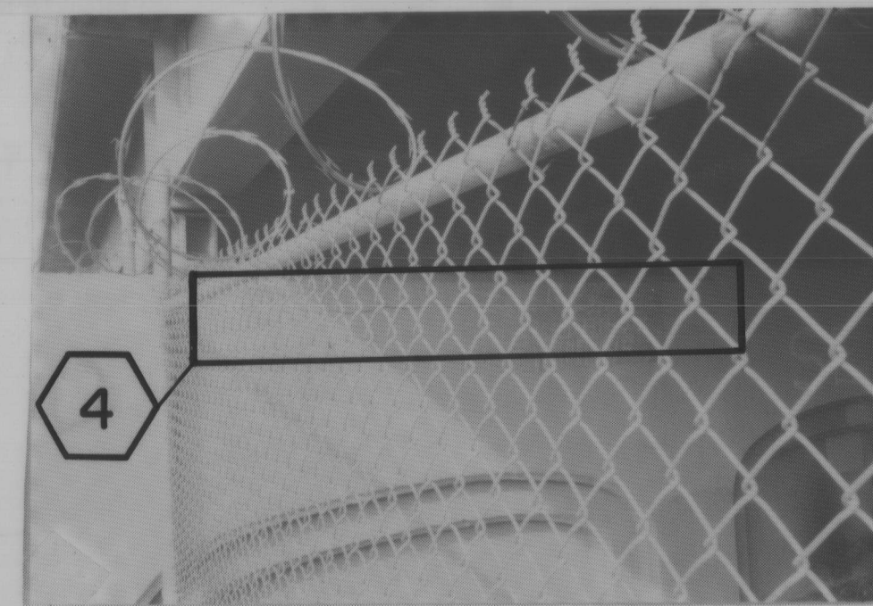
PHOTO N°3 PIER N°1 Between Southerly Beams
