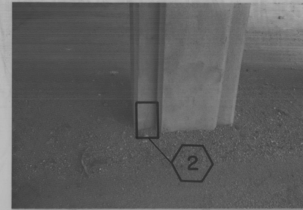
PHOTO N°9 PIER N°5 Eastside - 2 ND Column from Northend
