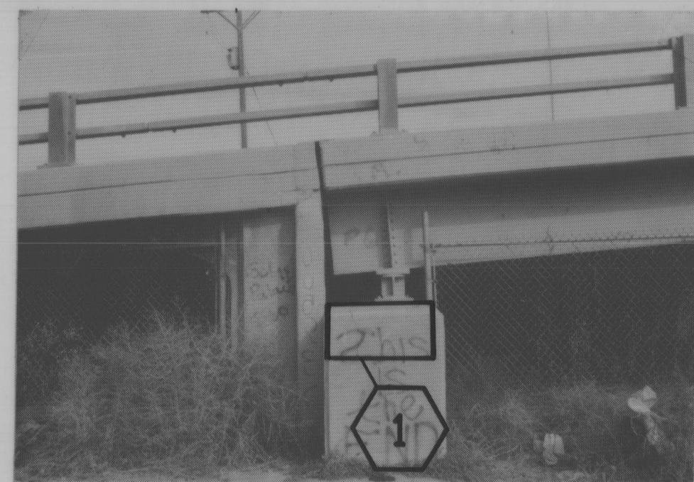
PHOTO N°1 ABUTMENT N°1 Southend
