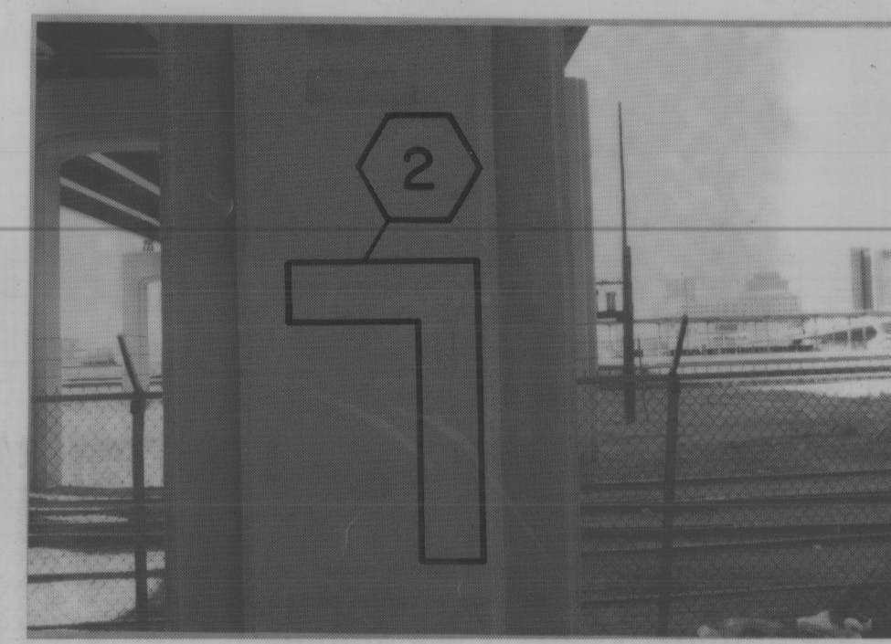
PHOTO N°14 PIER N°12 Eastside - North Column
