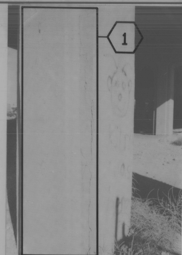
PHOTO Nº 17 PIER Nº 12 Westside - 2 ND Column from Southend
