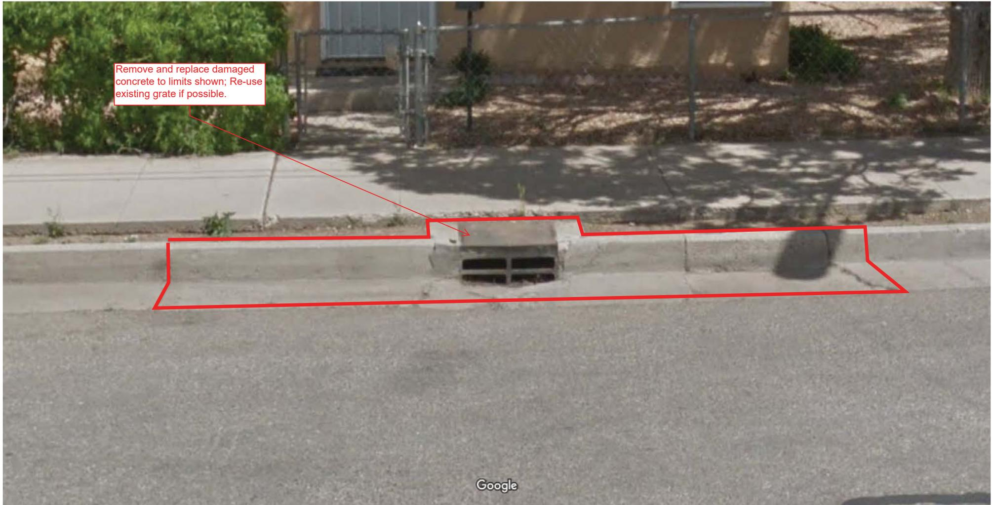
Remove and replace damaged concrete to limits shown; Re-use existing grate if possible.
