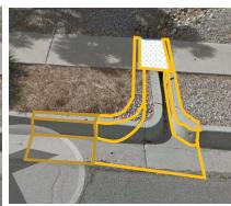
Placement — 1.0' sidewalk culvert – new curb
