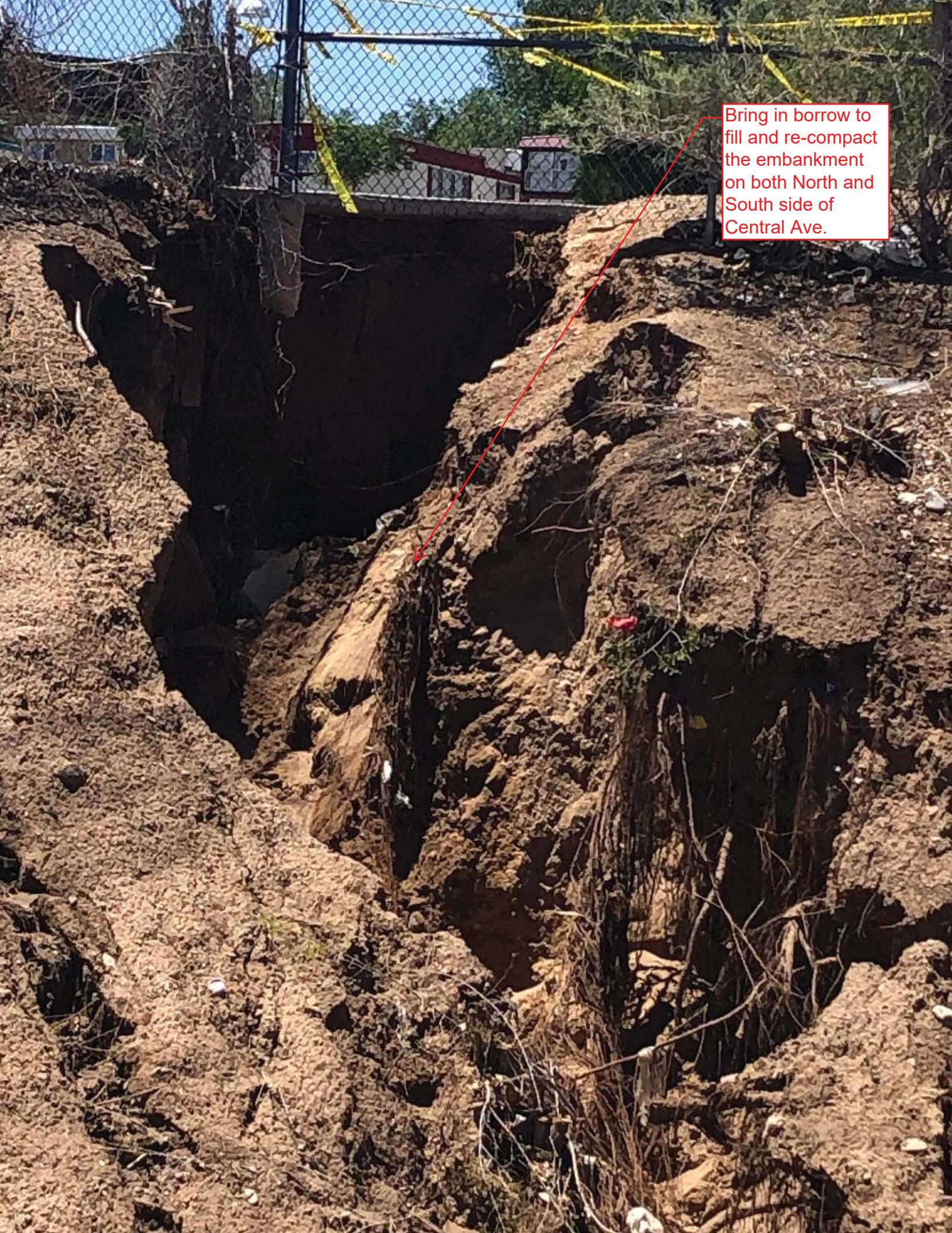
Bring in borrow to fill and re-compact the embankment on both North and South side of Central Ave.
