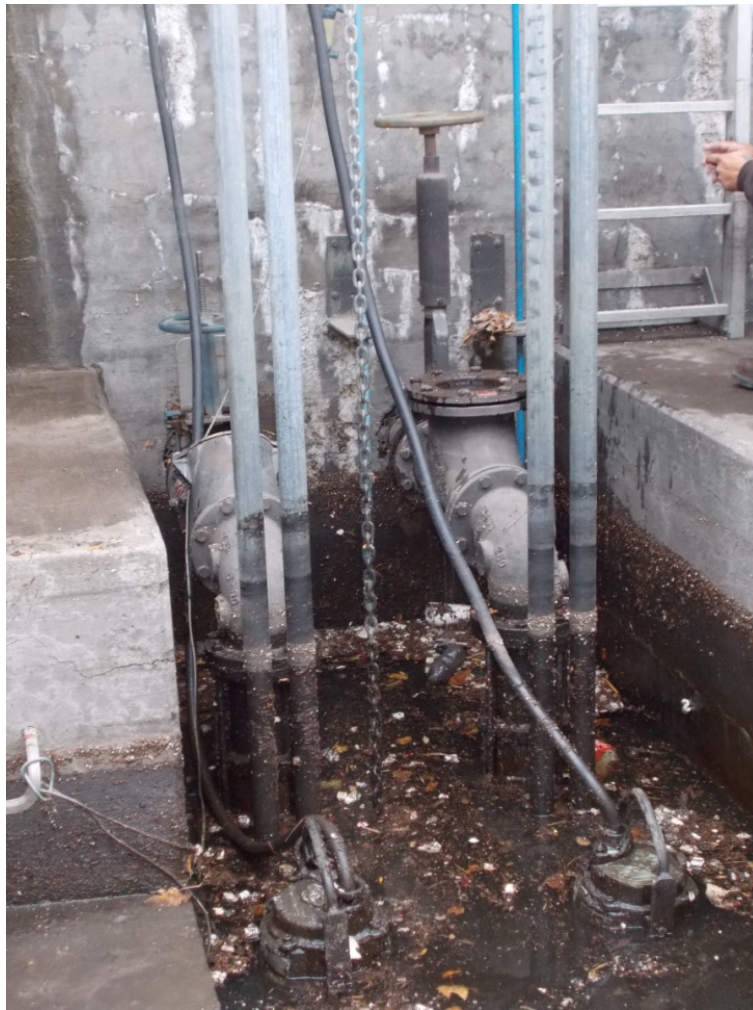
FIGURE 4-3 SUMP PUMPS AND VALVES
