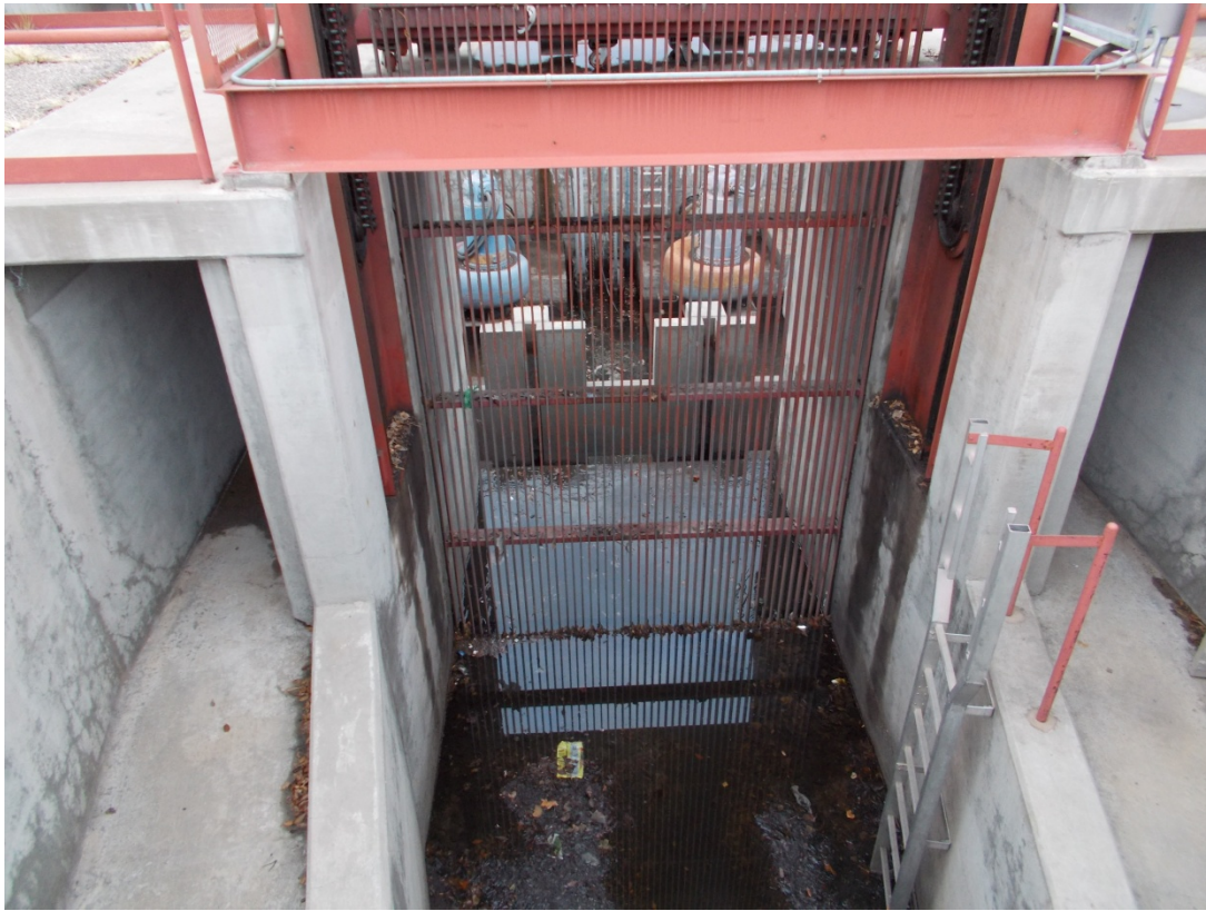
FIGURE 4-1 MECHANICAL BAR SCREEN AND OVERFLOW CHANNELS
