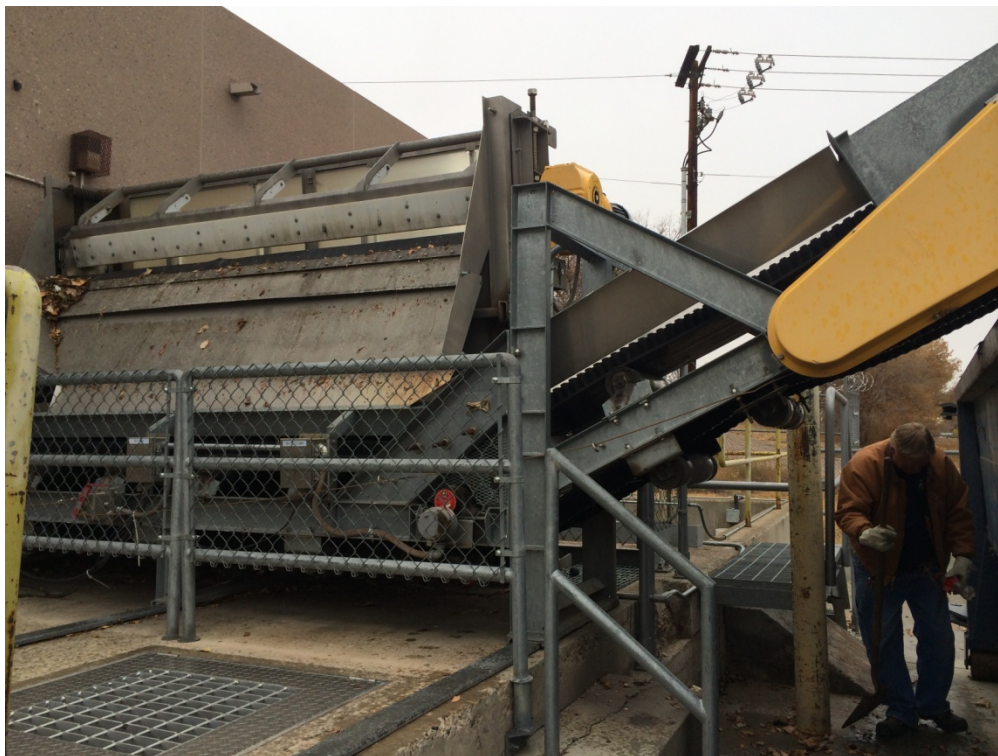
FIGURE 4-2 SCREENINGS CONVEYOR
