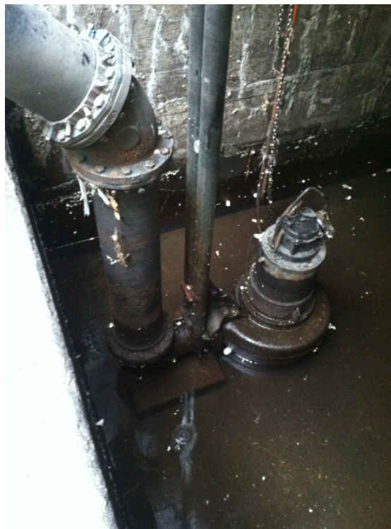
FIGURE 4-4 SUMP PUMP
