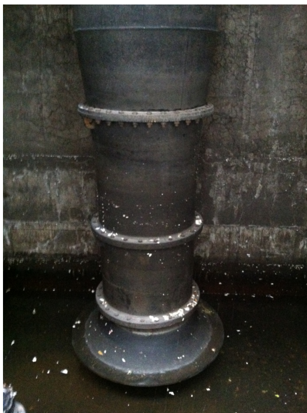
FIGURE 4-3 LIFT PUMPS
