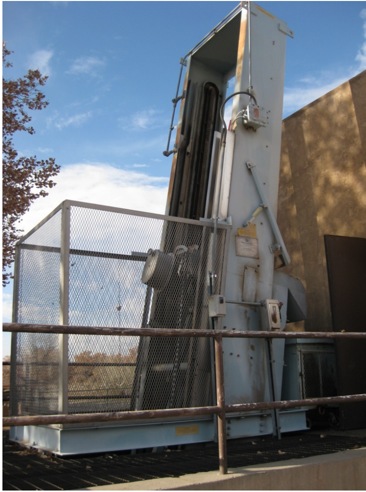
FIGURE 4-1 MECHANICAL BAR SCREEN
