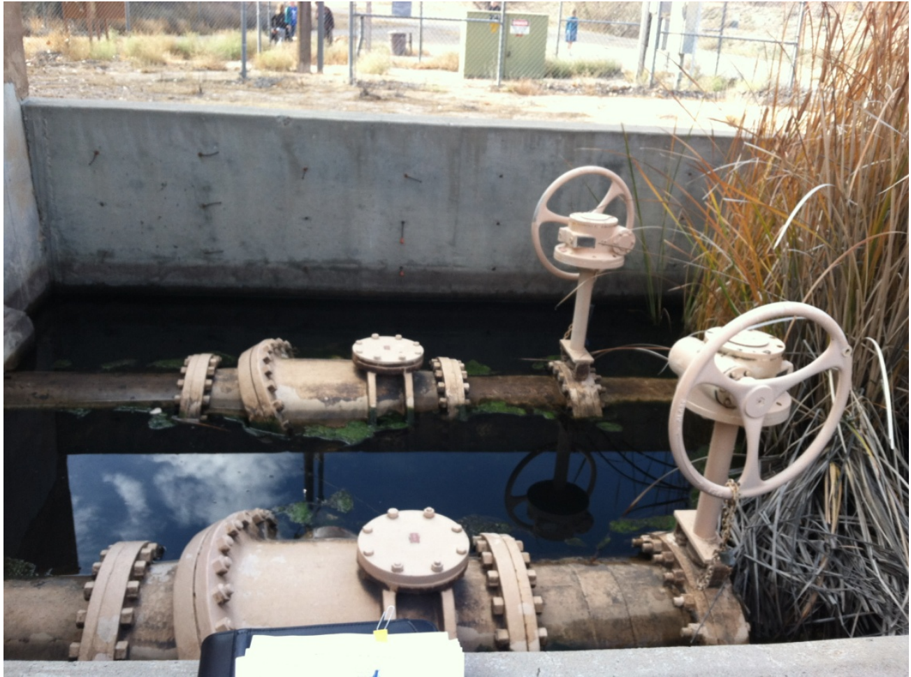
FIGURE 4-3 VALVE VAULT
