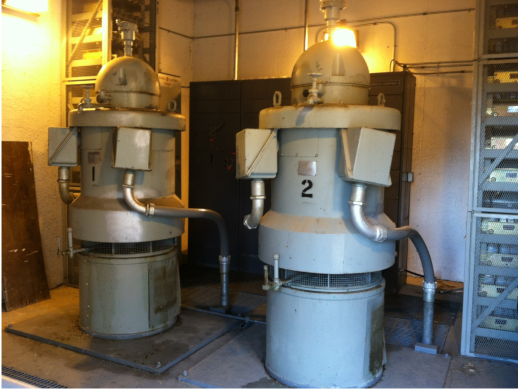
FIGURE 4-2 LIFT PUMP MOTORS
