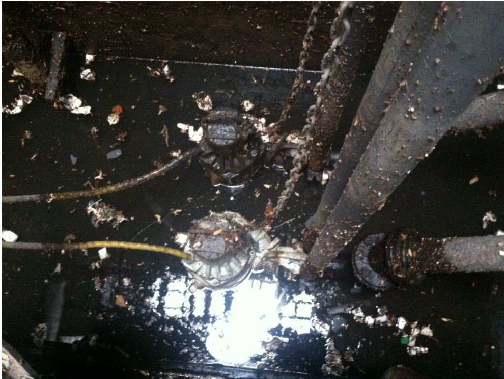
FIGURE 4-3 SUMP PUMPS
