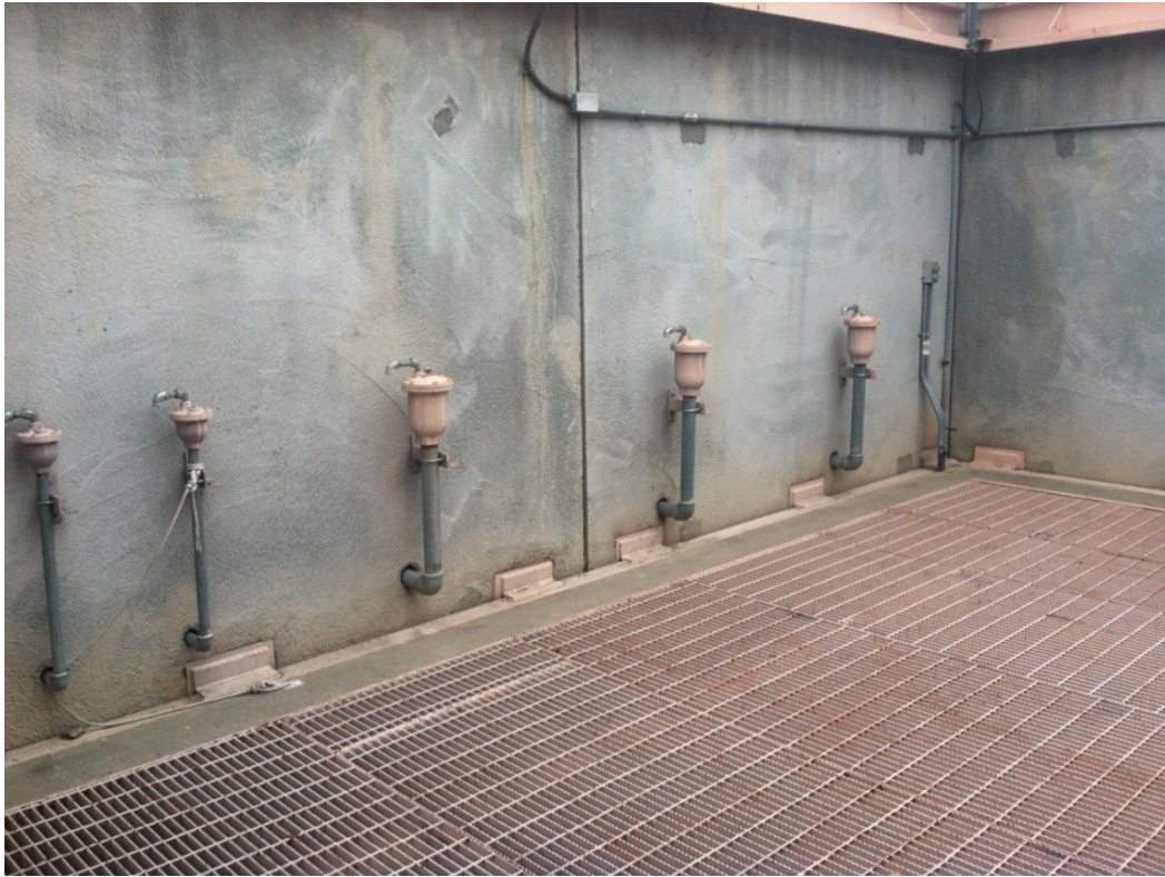
FIGURE 4-4 AIR RELIEF VALVES
