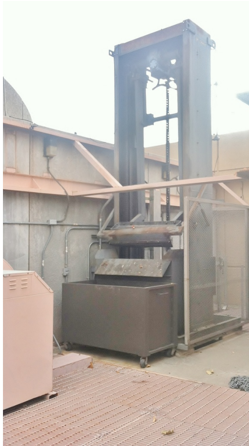
FIGURE 4-1 MECHANICAL BAR SCREEN
