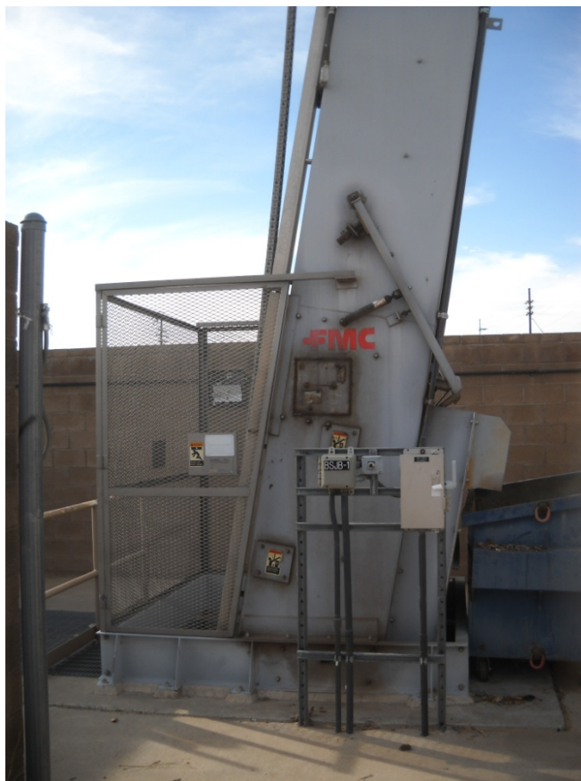
FIGURE 4-1 MECHANICAL BAR SCREEN
