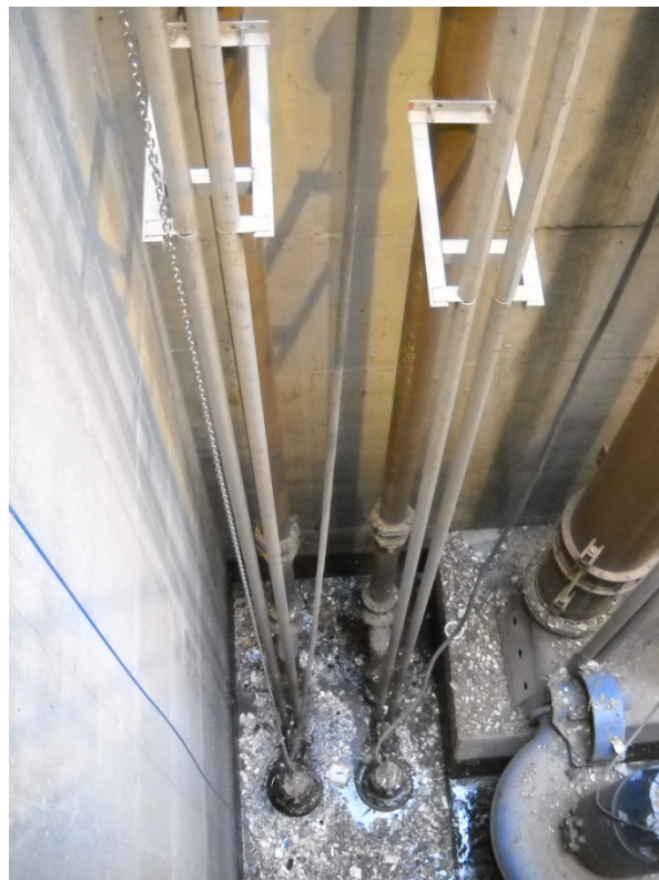
FIGURE 4-3 SUMP PUMPS
