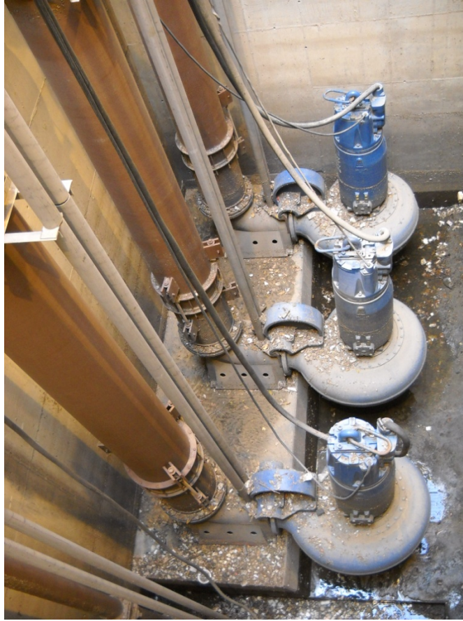
FIGURE 4-2 LIFT PUMPS
