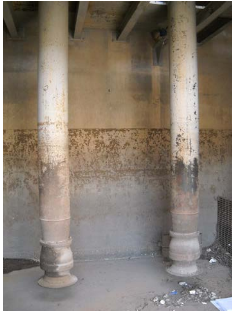
FIGURE 4-3 LIFT PUMP INTAKES
