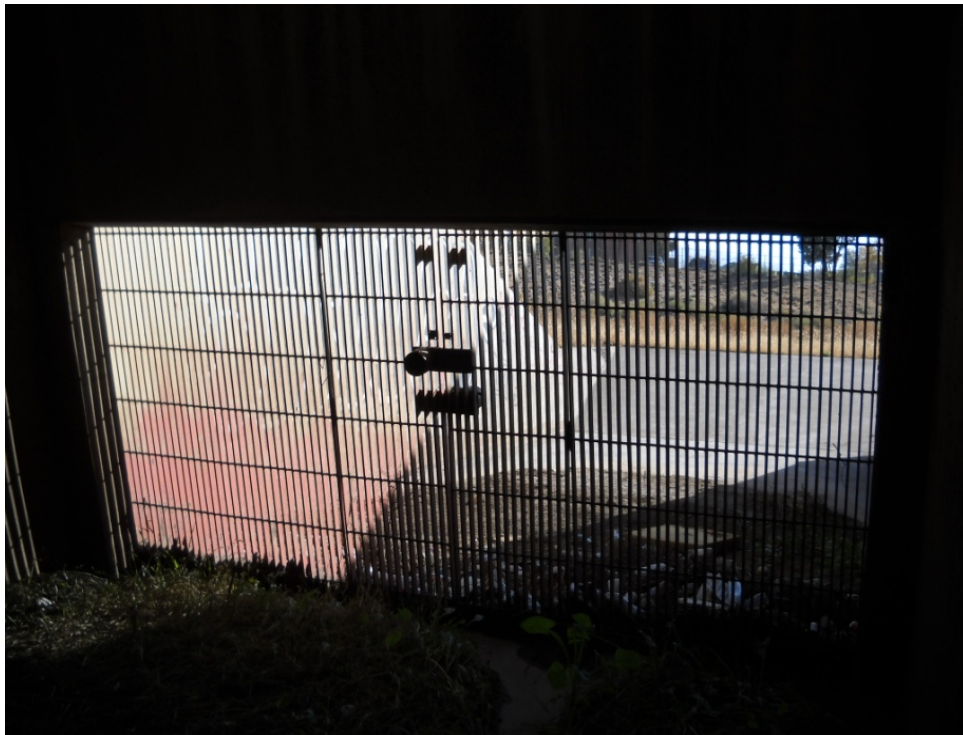
FIGURE 4-1 FIXED BAR SCREEN
