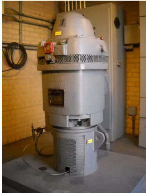
FIGURE 4-2 LIFT PUMP MOTOR
