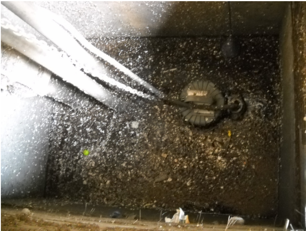
FIGURE 4-4 SUMP PUMP
