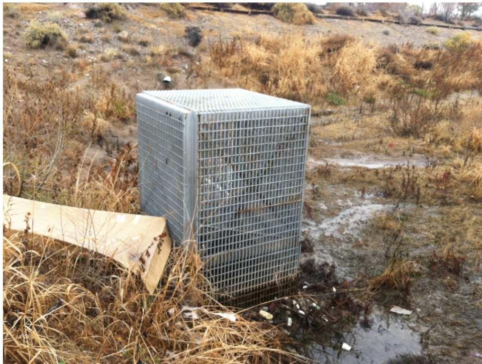
FIGURE 4-1 BAR SCREEN CAGE
