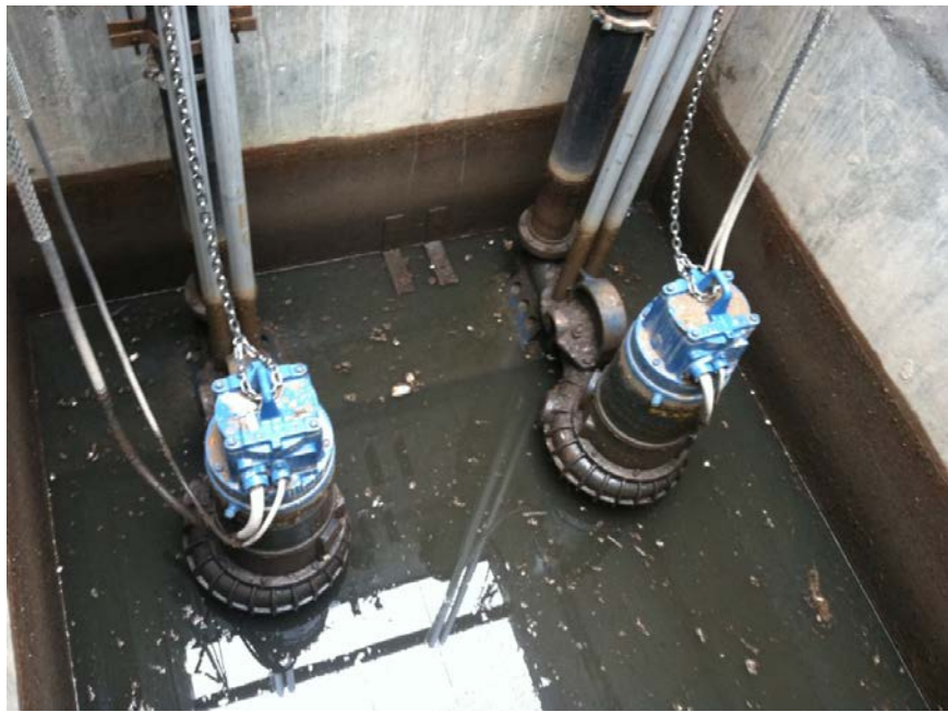
FIGURE 4-2 WET WELL AND LIFT PUMPS
