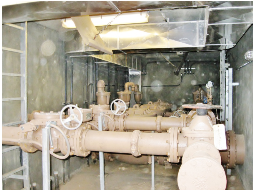
FIGURE 4-4 VALVE VAULT
