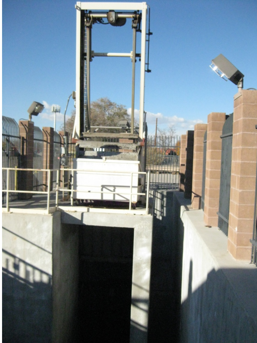
FIGURE 4-1 MECHANICAL BAR SCREEN
