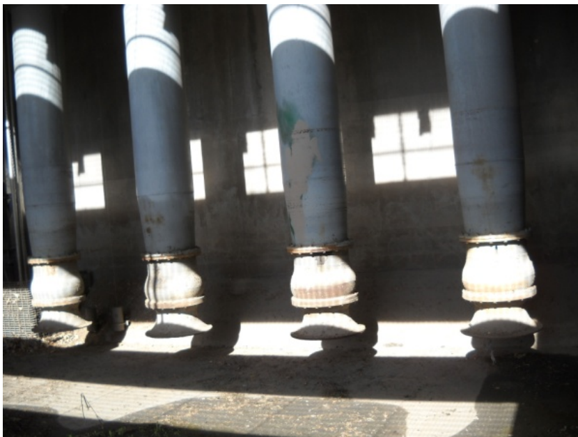
FIGURE 4-2 LIFT PUMP MOTORS AND INTAKES
