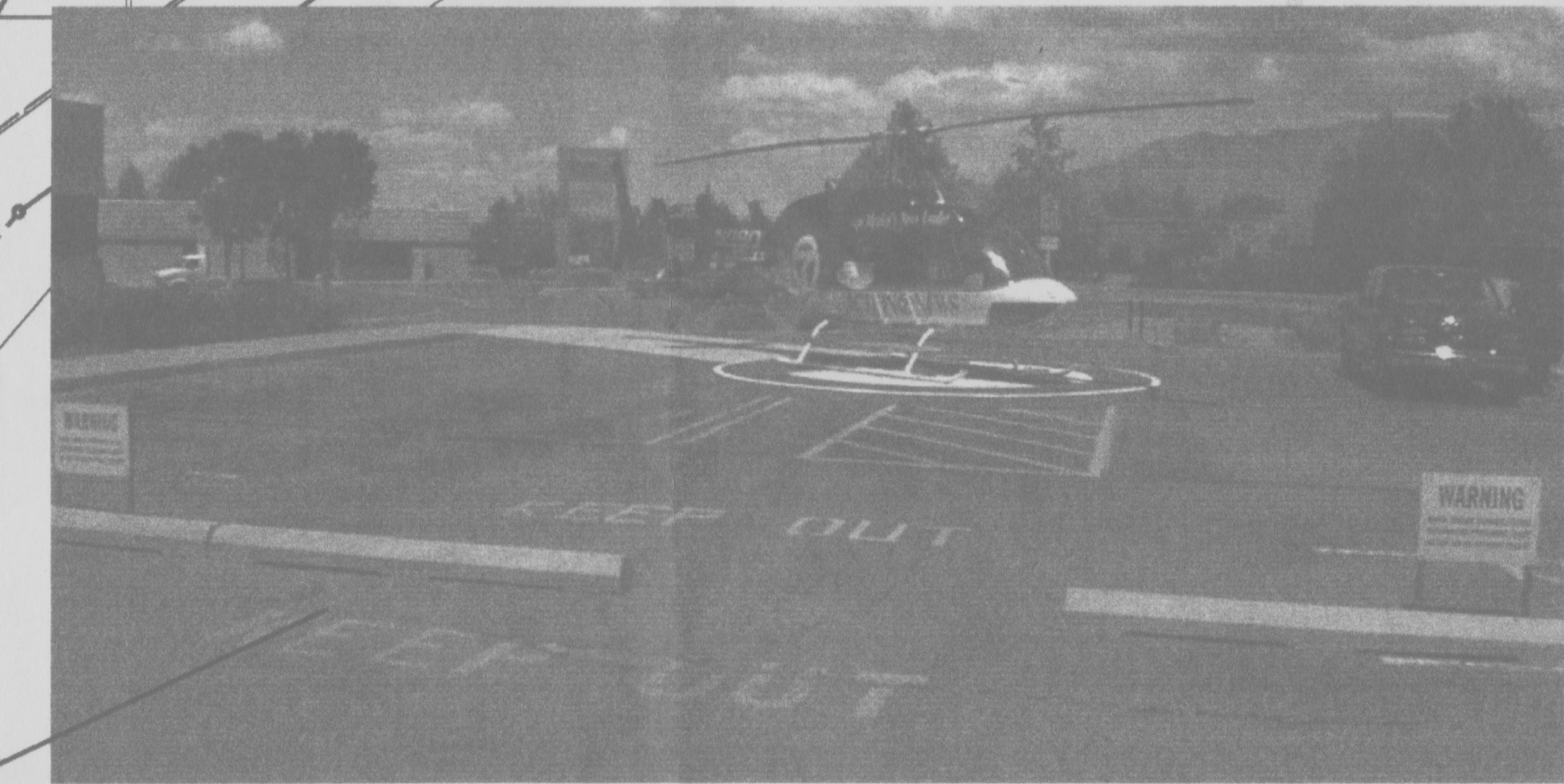
VIEW OF HELIPAD LOOKING EAST
