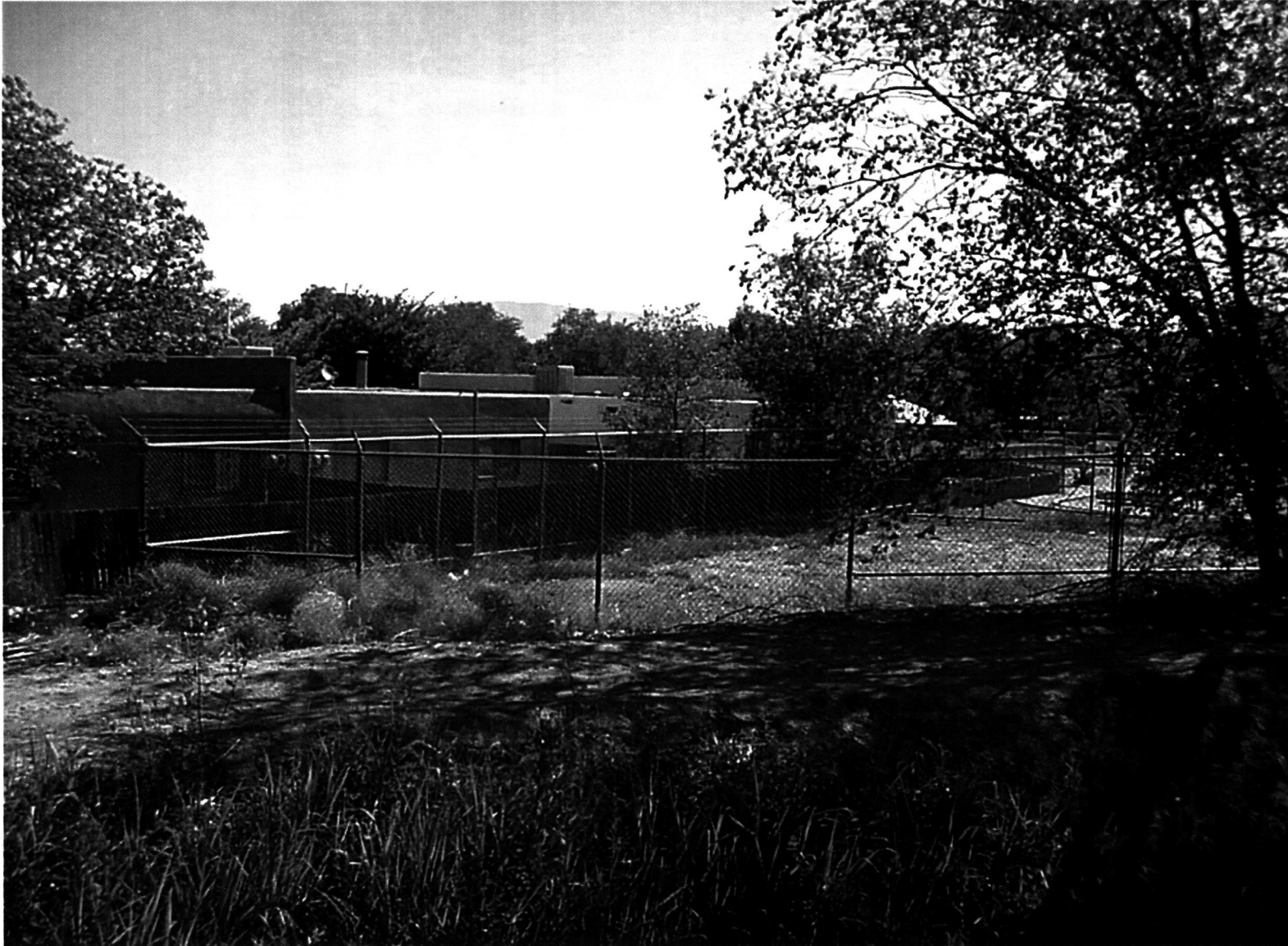
LOOKING NORTHEAST FROM WEST SIDE OF SITE
