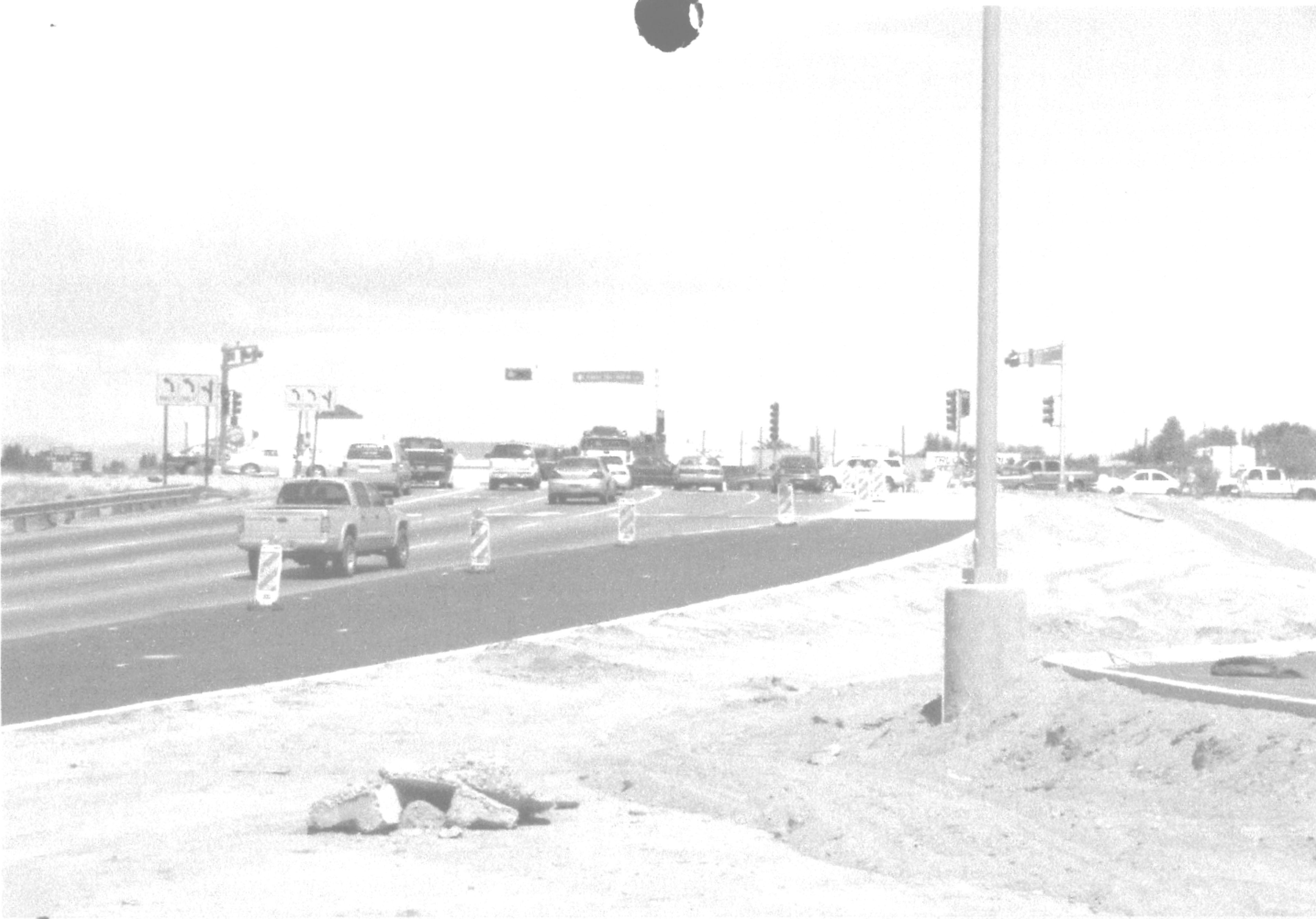
FRONTAGE ROAD WIDENING
