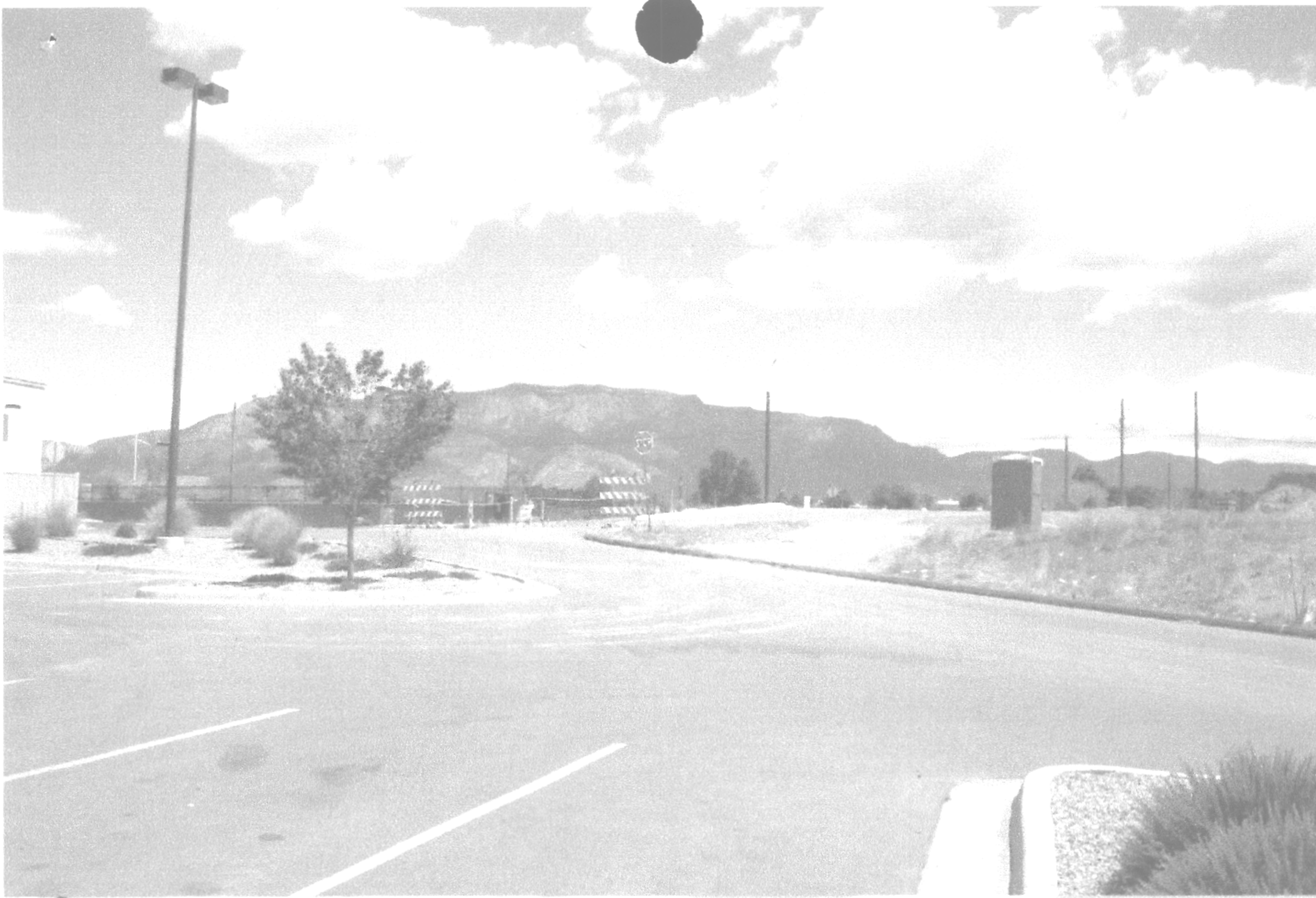
SAN PEDRO RECONSTRUCTION (from inside site)
