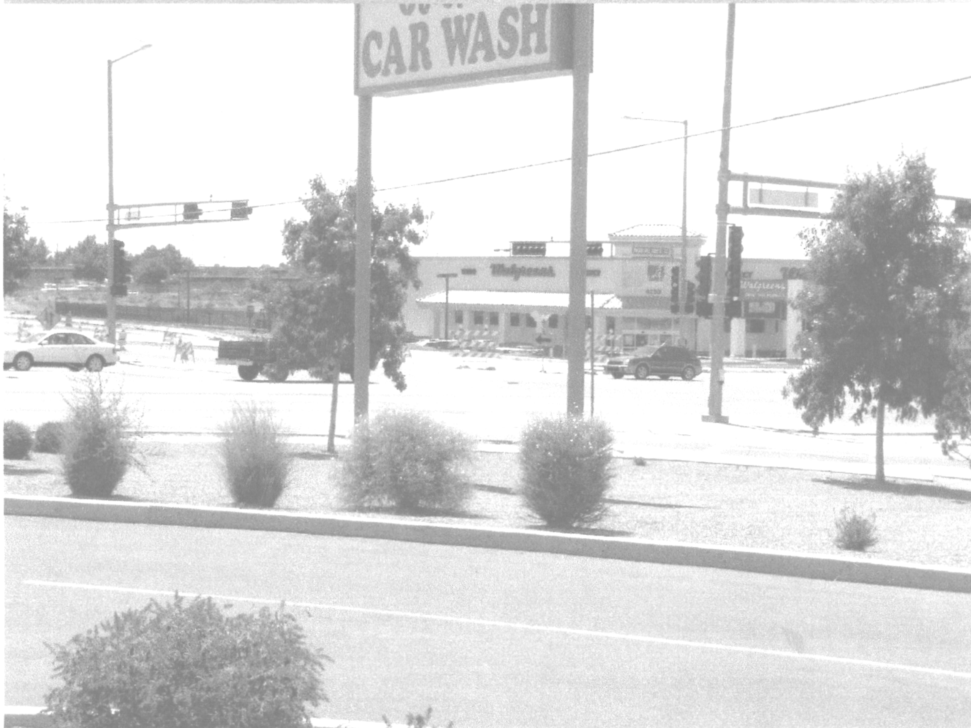
SAN PEDRO RECONSTRUCTION (from NE corner of PDN intersection)
