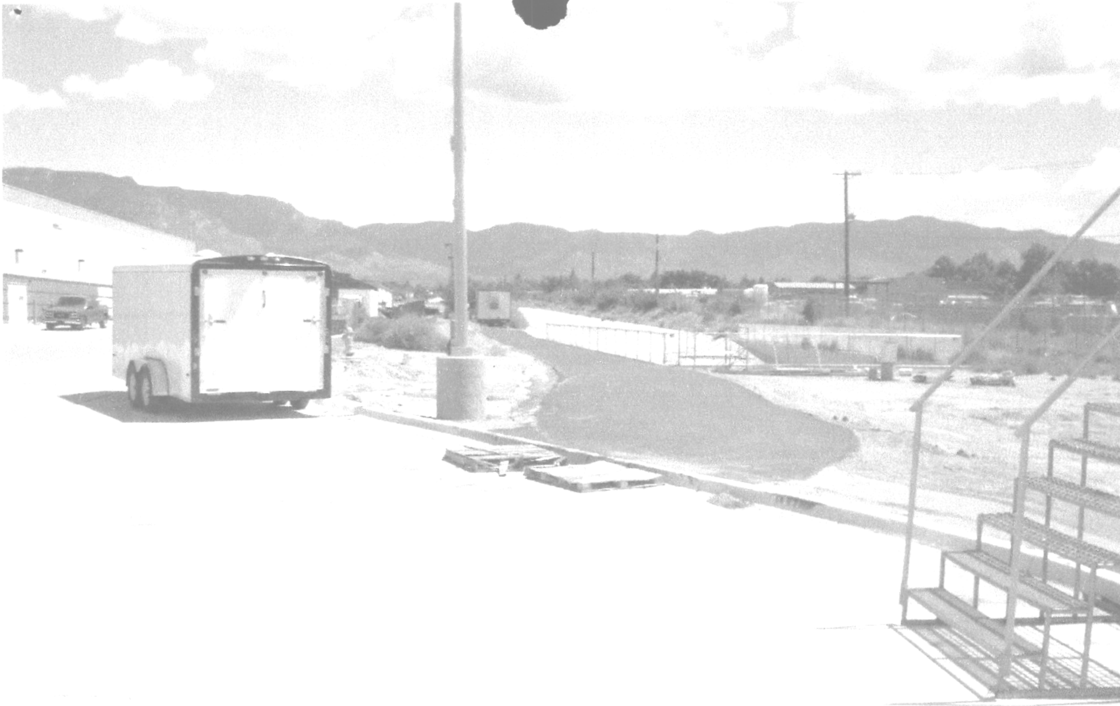
Existing Trail Ends Under Construction Trailer
