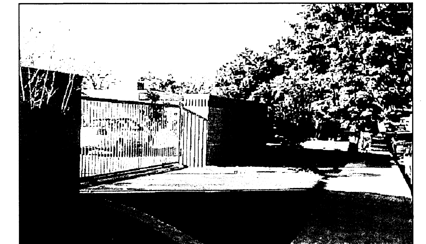
"A" PHOTOGRAPH SHOWING THE PROPOSED TYPE OF GATE & CONCRETE MASONRY BLOCK WALL (NOTE: THE HEIGHT OF THE CONCRETE MASONRY BLOCK WALL IS TO BE 8'-0" ALONG THE NORTH AND EAST SIDES. THE HEIGHT WILL BE 7'-2" ALONG VERMONT STREET TO MATCH THE EXISTING WALL TO THE SOUTH. THE COLOR OF BLOCK IS TO BE "CREGG TAN" FROM CSR. (THIS COLOR IS A LIGHT EARTH TONE BROWN.) THE FLUTTED CAP WILL BE INSTALLED ON THE WALL ALONG VERMONT ST. ONLY.)
