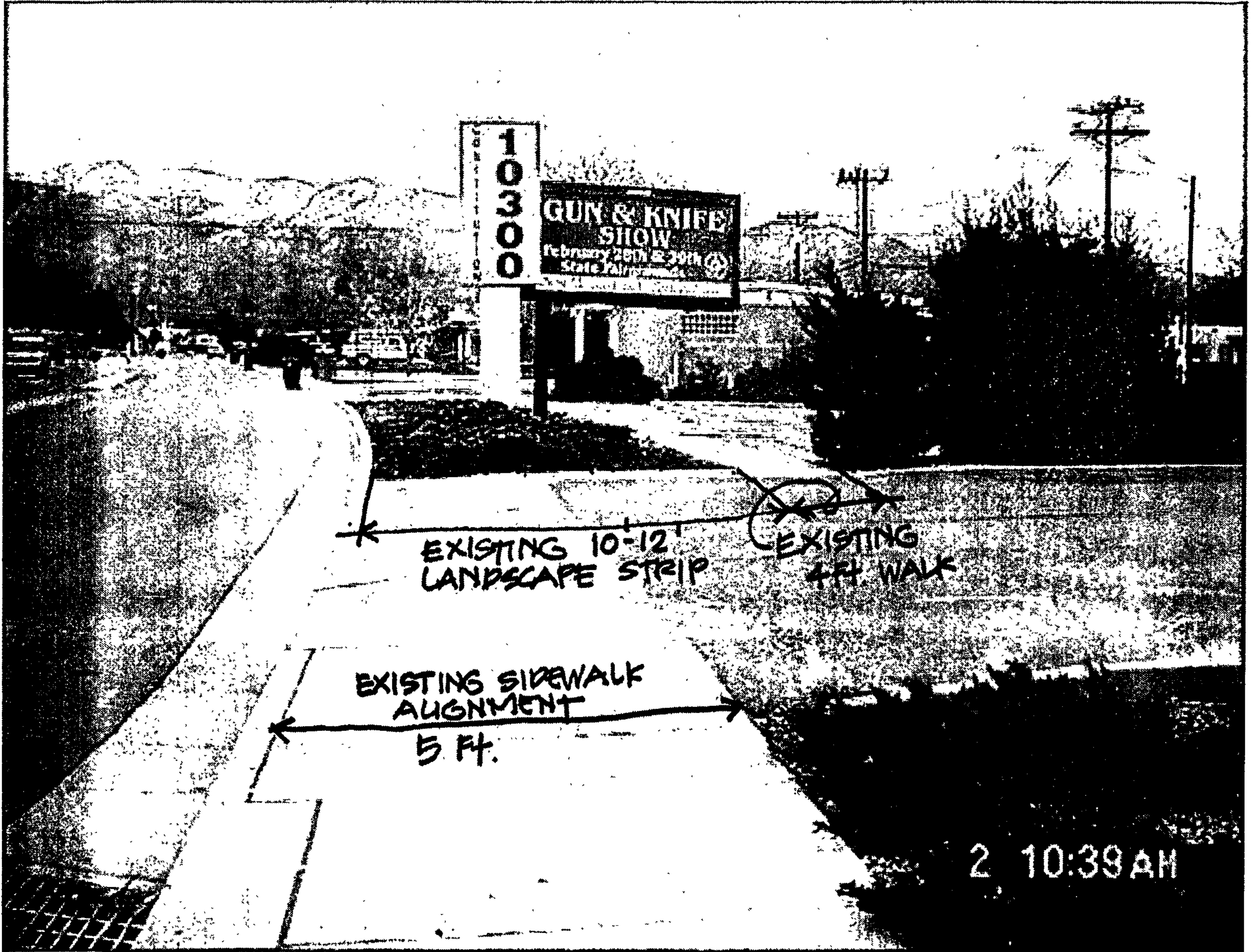
EXISTING SIDEWALK - VIEW TO EAST
