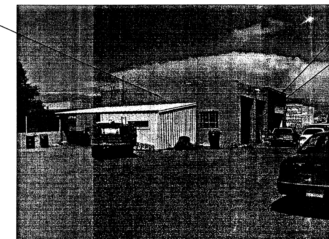
SIDE ELEVATION: EXISTING GARAGE ON SU-1 PORTION 16' TO ROOF OF CMU PORTION OF GARAGE (WEST FACE)
