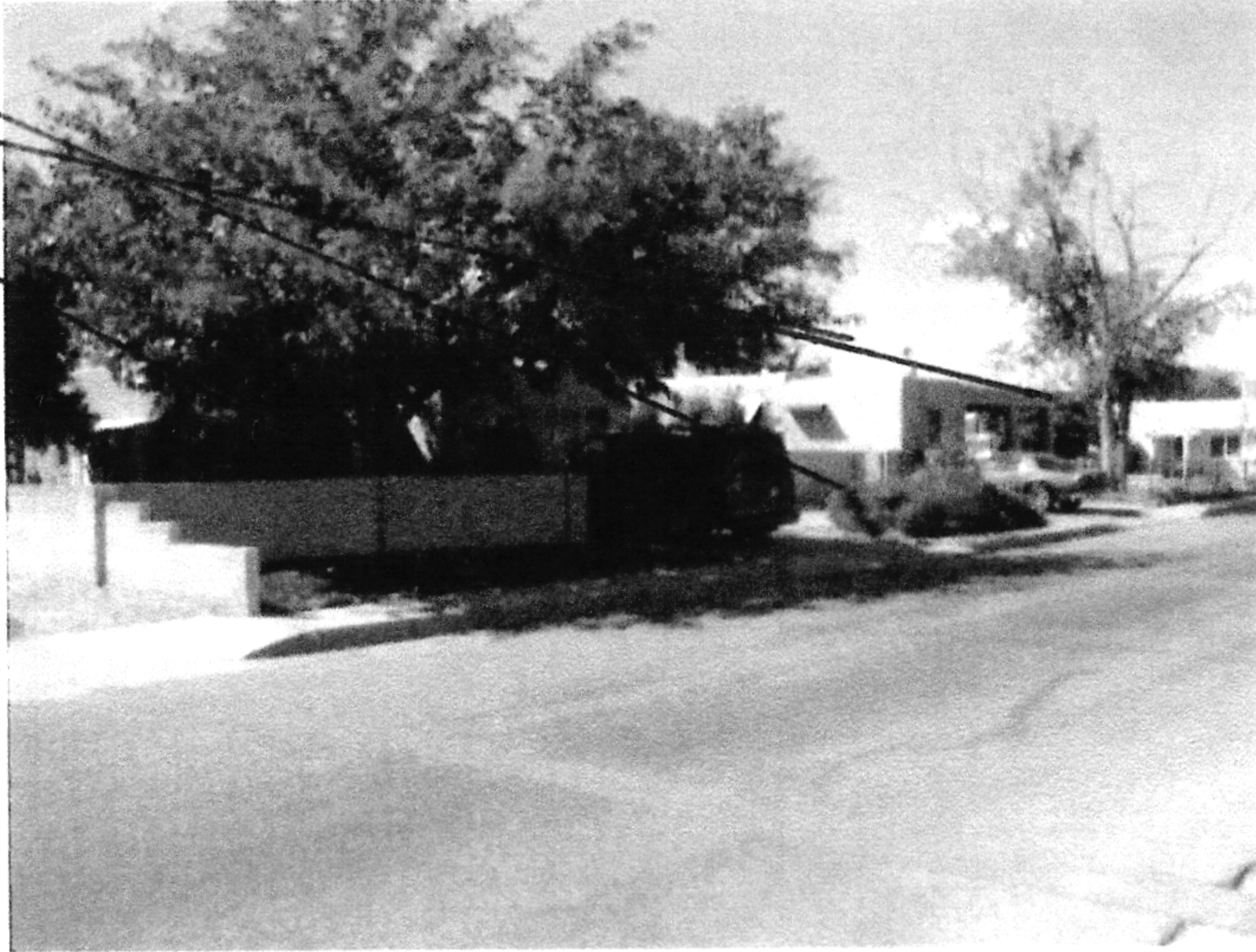
1211 and 1215 Madeira, and 5320 Granite
