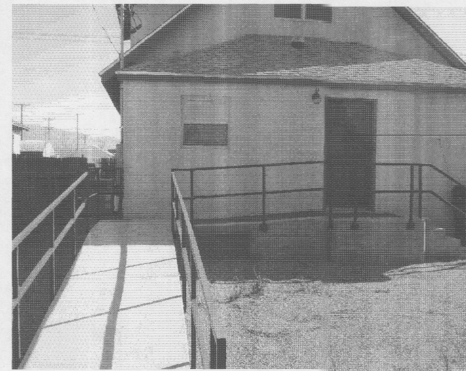
WEST ELEVATION SHOWING RAMP
