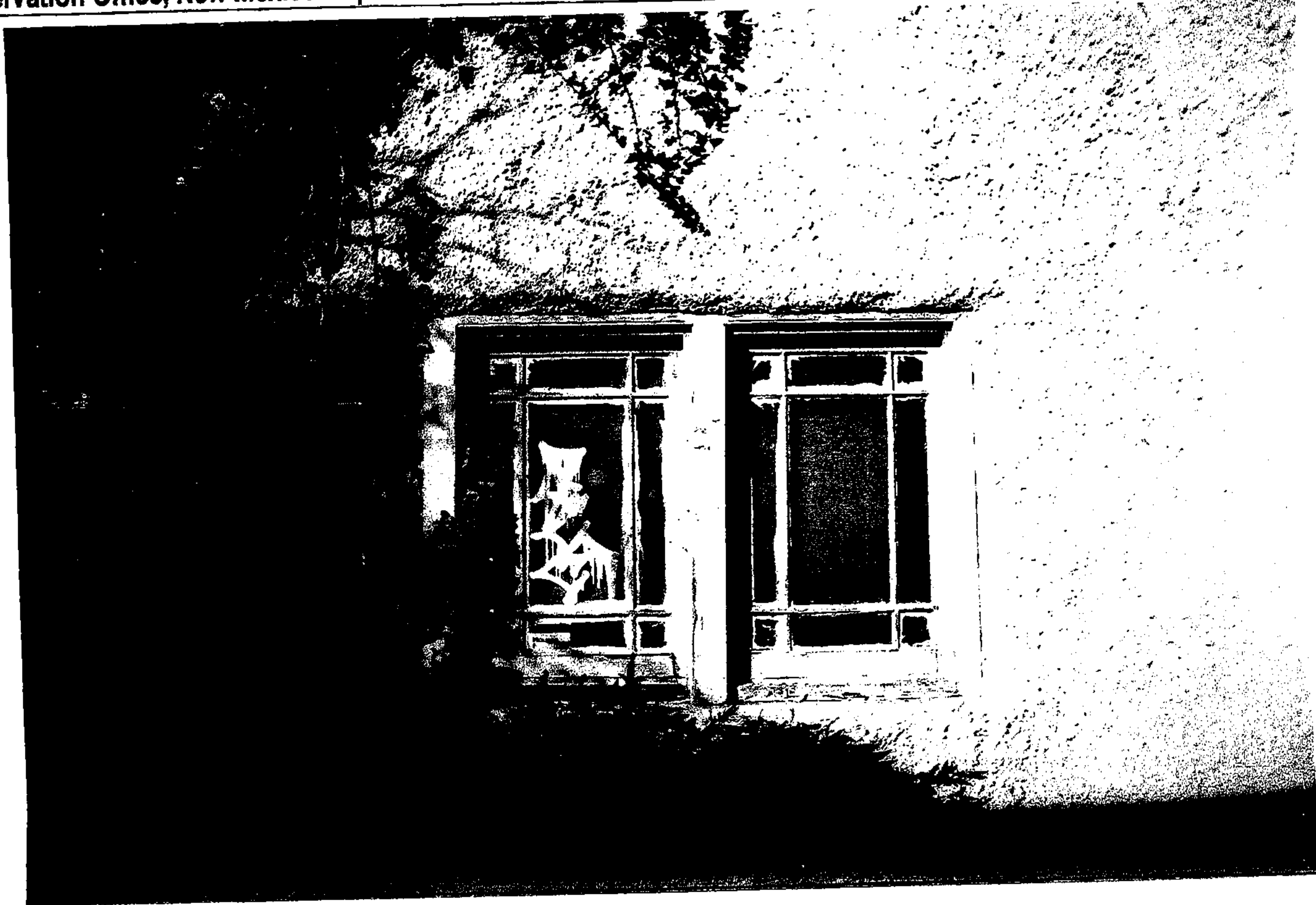
WINDOW, S ELEV., CENTER. OTHER WINDOWS HAVE NO MUNTINS
