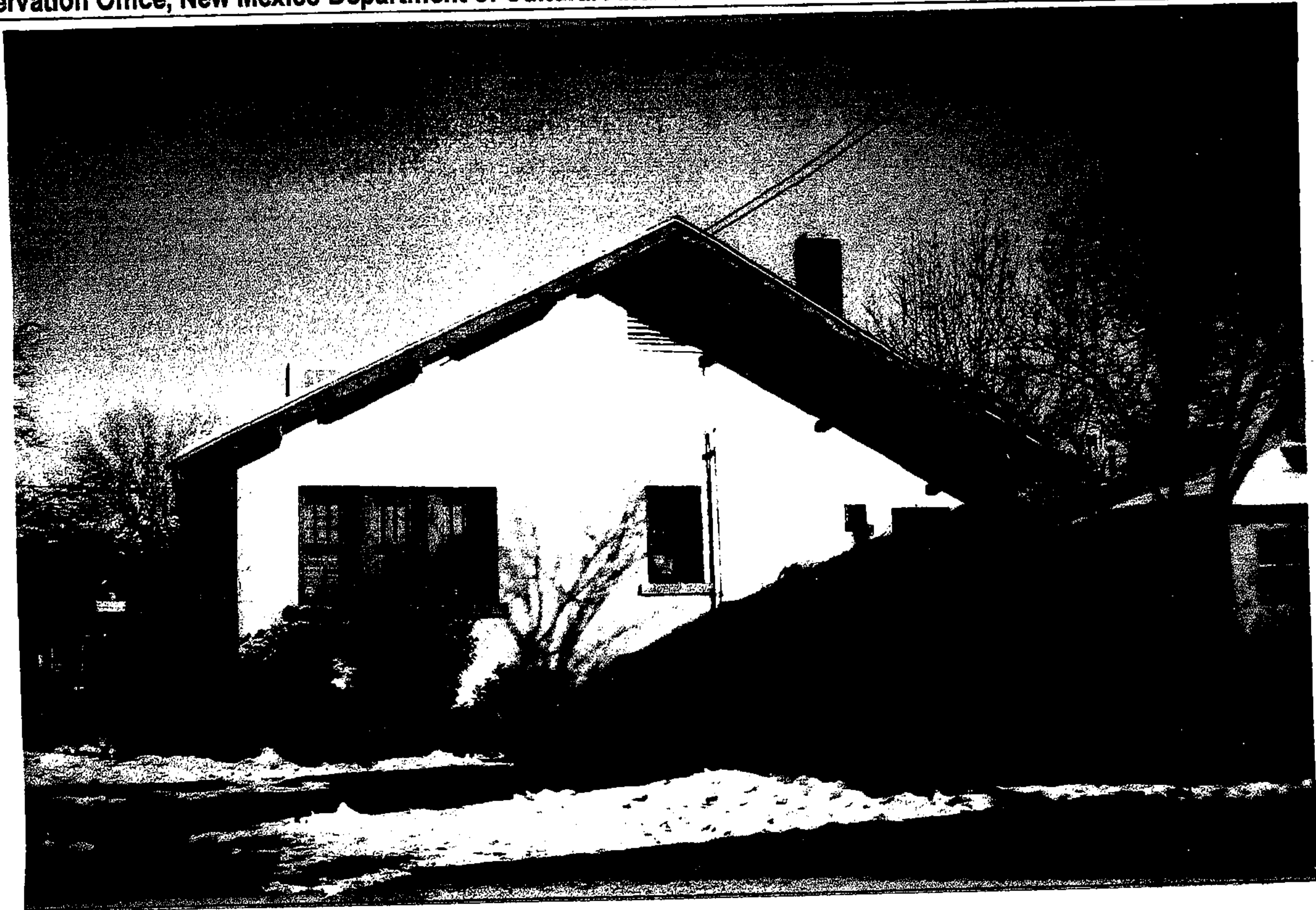
WEST (REAR) ELEVATION SHOWING EXPOSED & PROTRUDING PURLINS - ABOUT 6" X 6"
