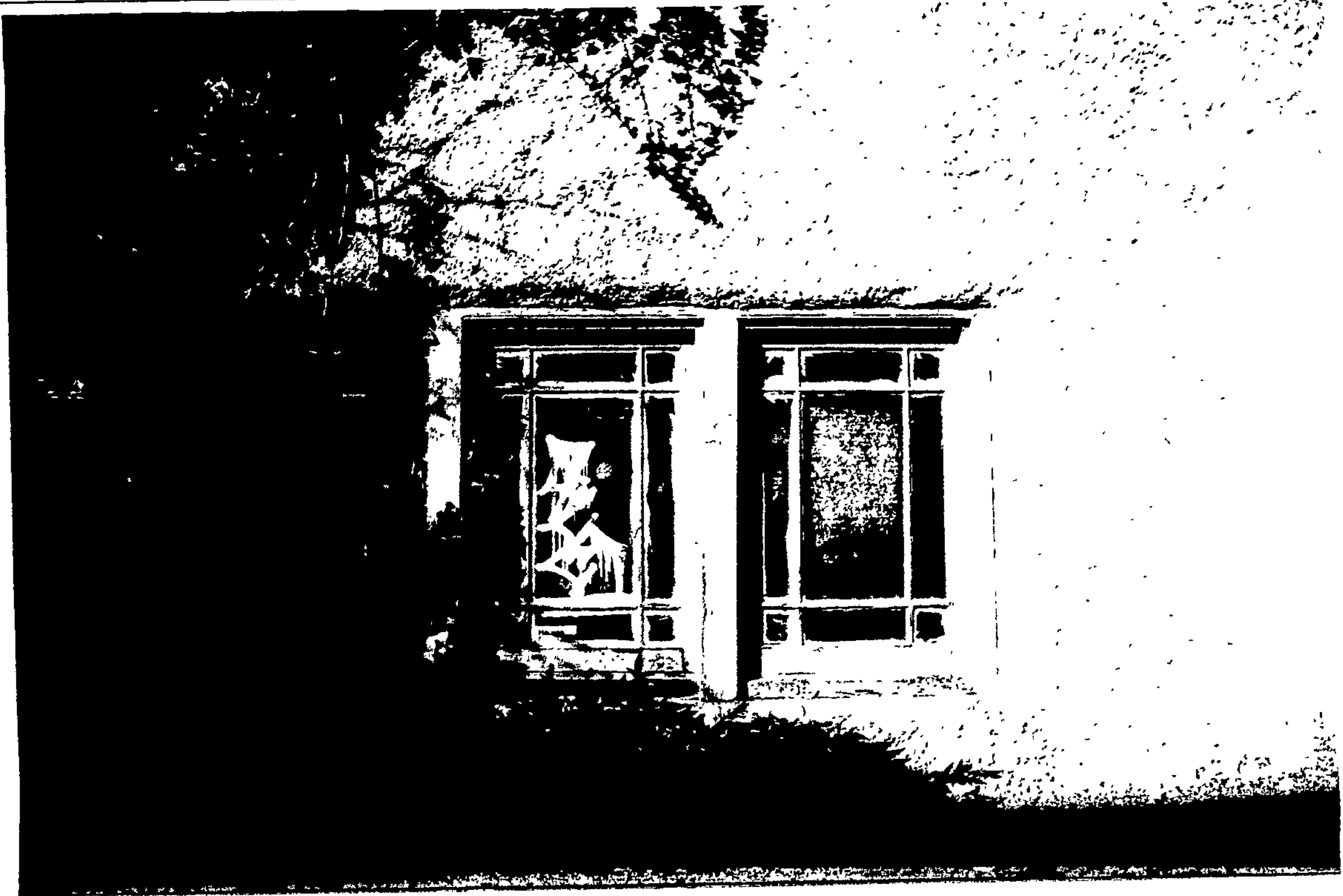
WINDOW, S ELEV., CENTER. OTHER WINDOWS HAVE NO MUNTINS
