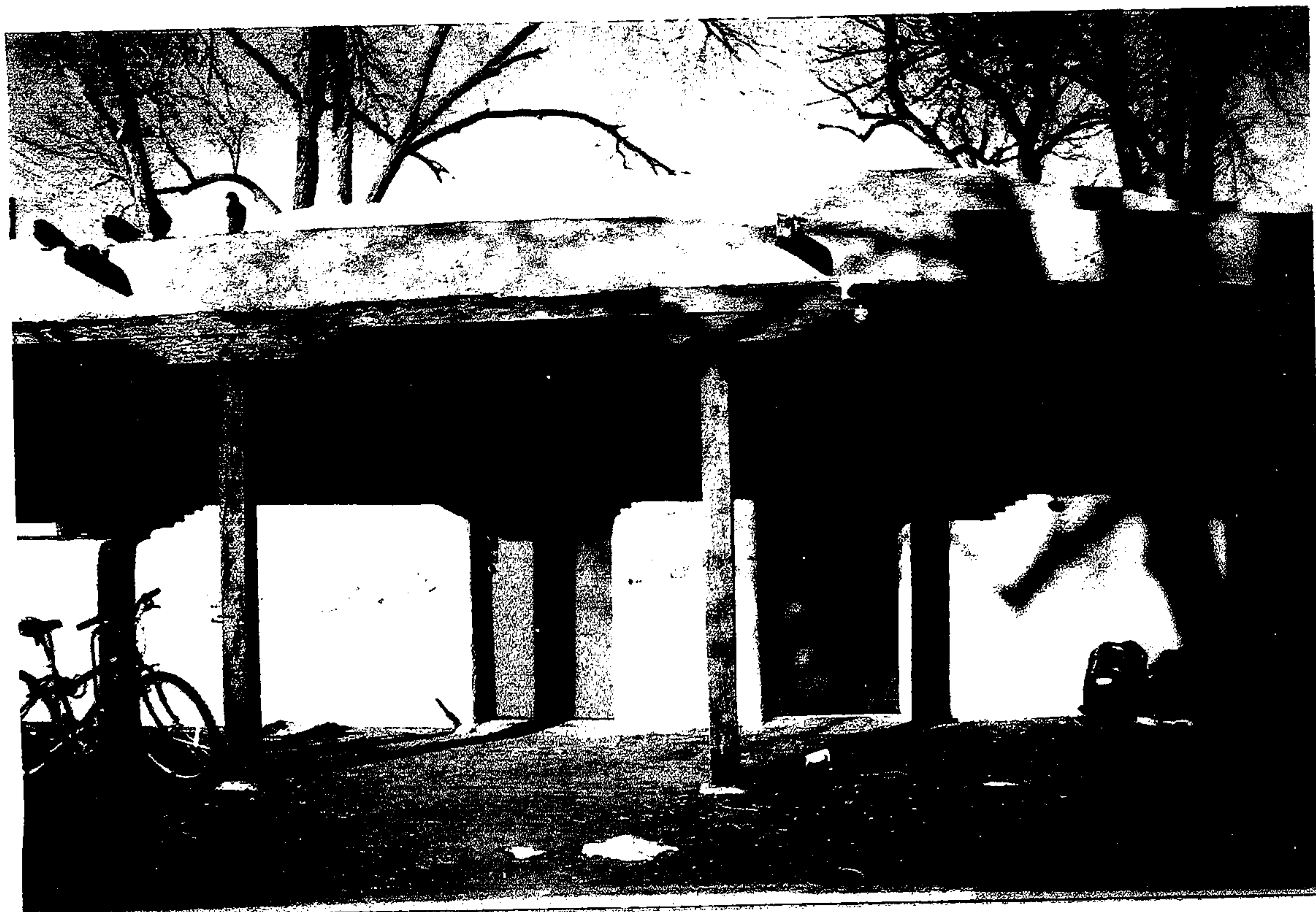
CLOSE-UP OF CORBELS & POSTS OF APT. PORTAL
