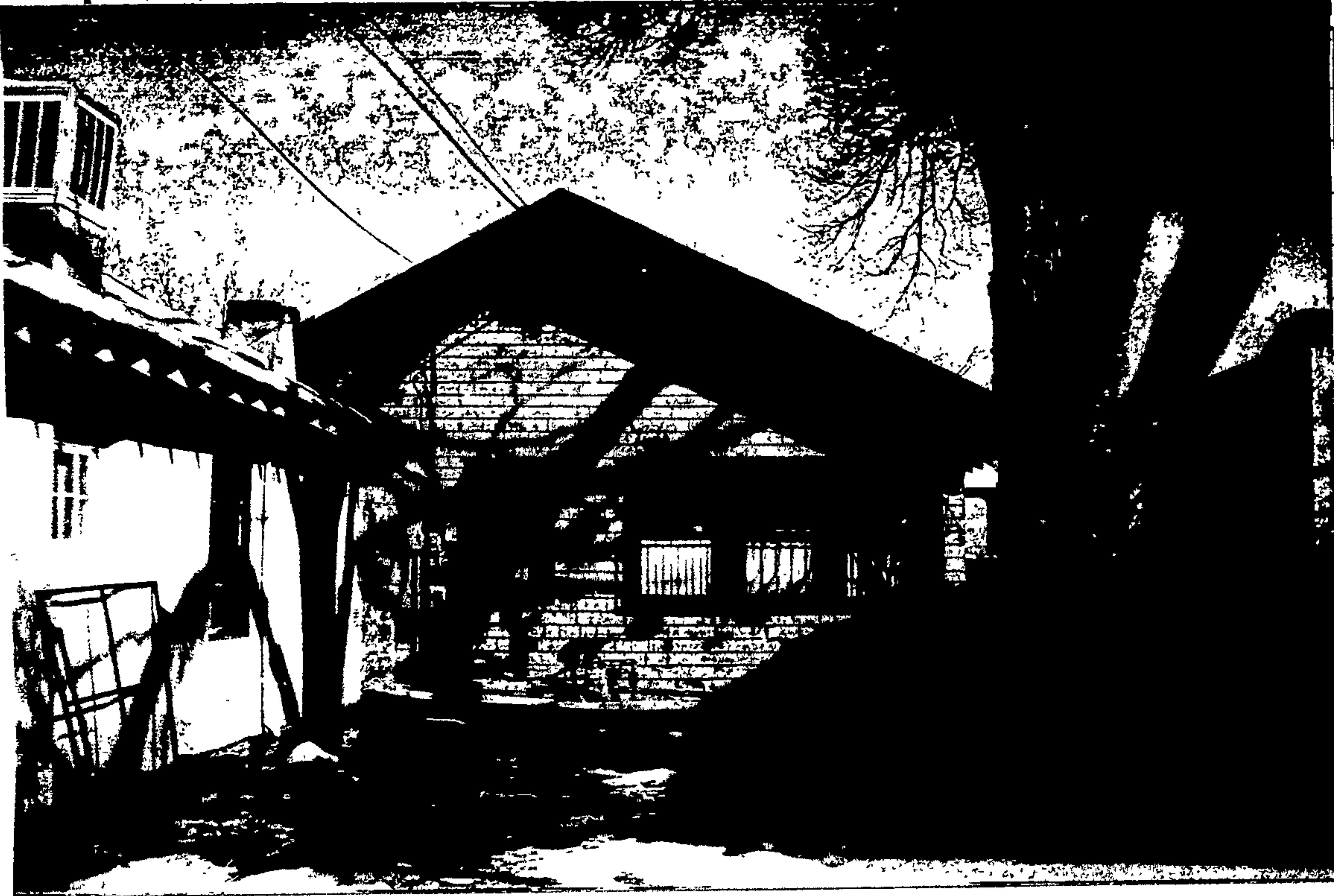
WEST (REAR) ELEVATION SHOWING WOOD SHINGLED SIDING
