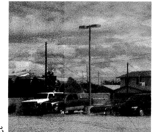
EXISTING PARKING LIGHT see note D on sheet AS-1 and L-1
