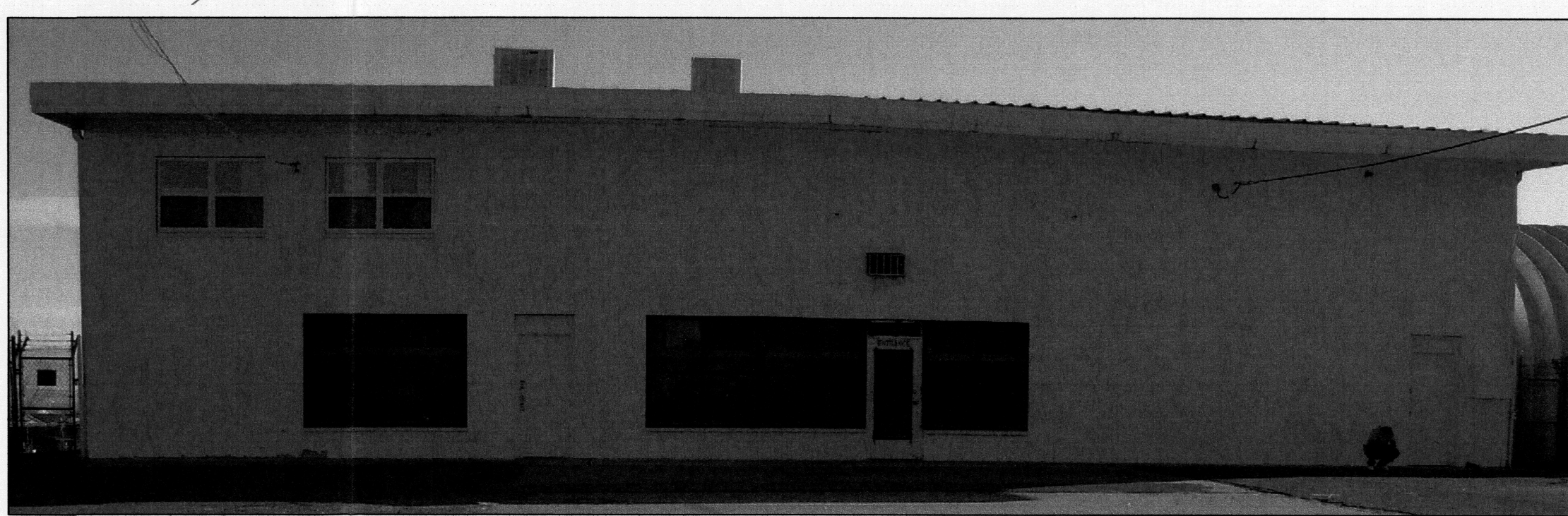
EXISTING WHITE BUILDING TO REMAIN
