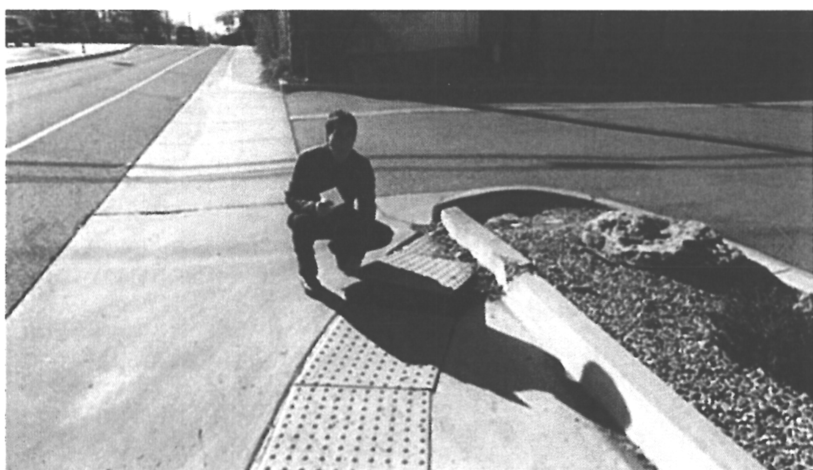
Photo 2e & 2f, Carlisle west side with station driveway
