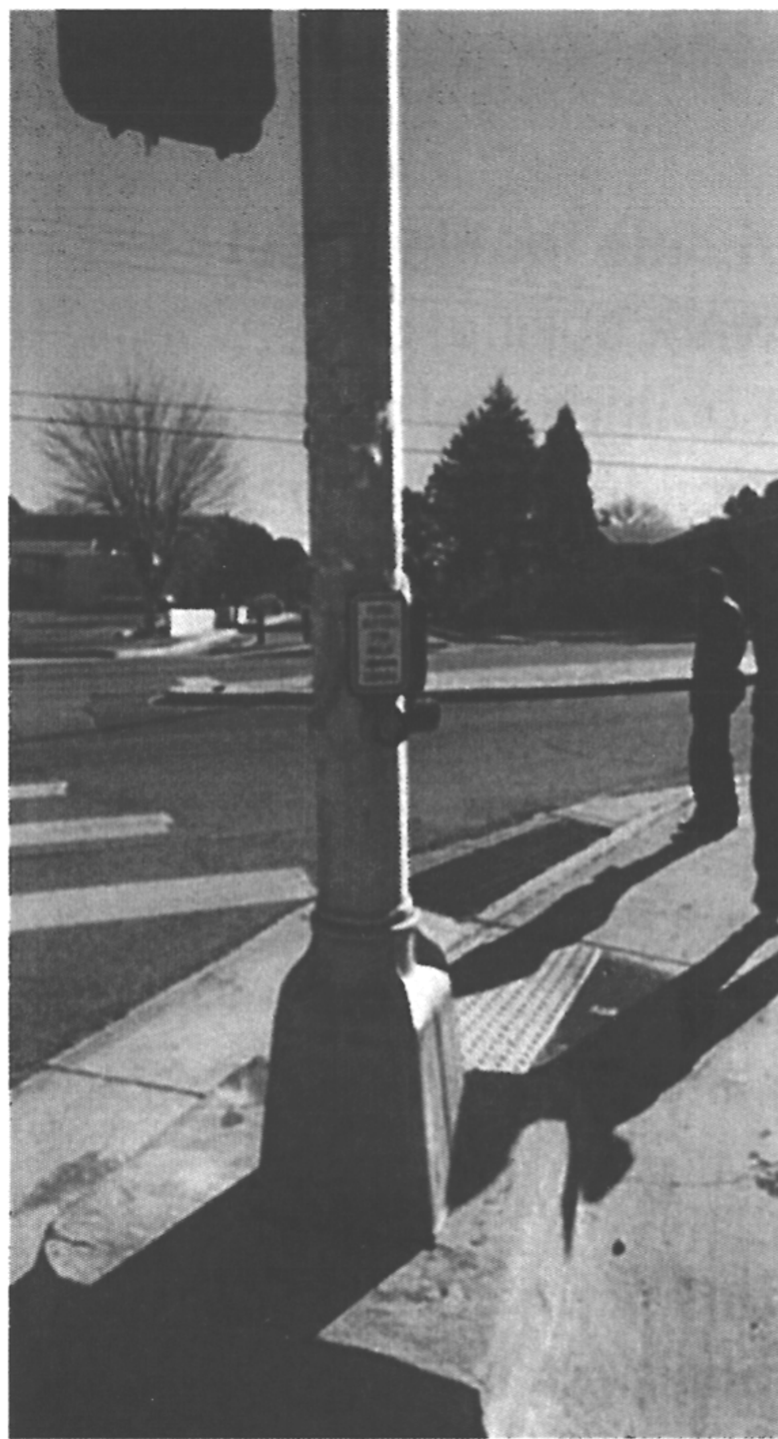
Photo 1e & 1f, signal light at SW corner of Constitution and Carlisle
