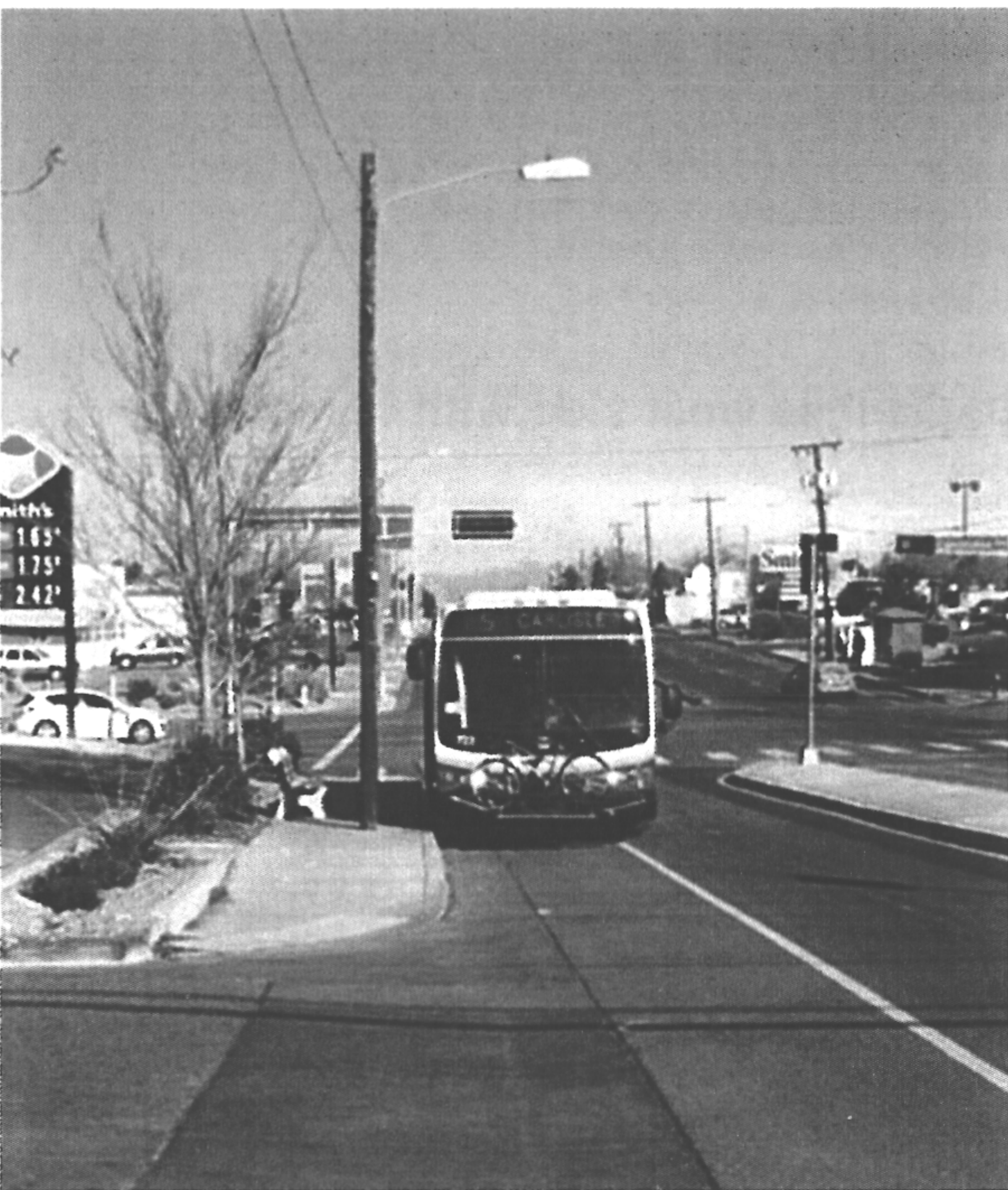
Photo 2b, BUS STOP, Carlisle west side looking north toward Constitution intersection
