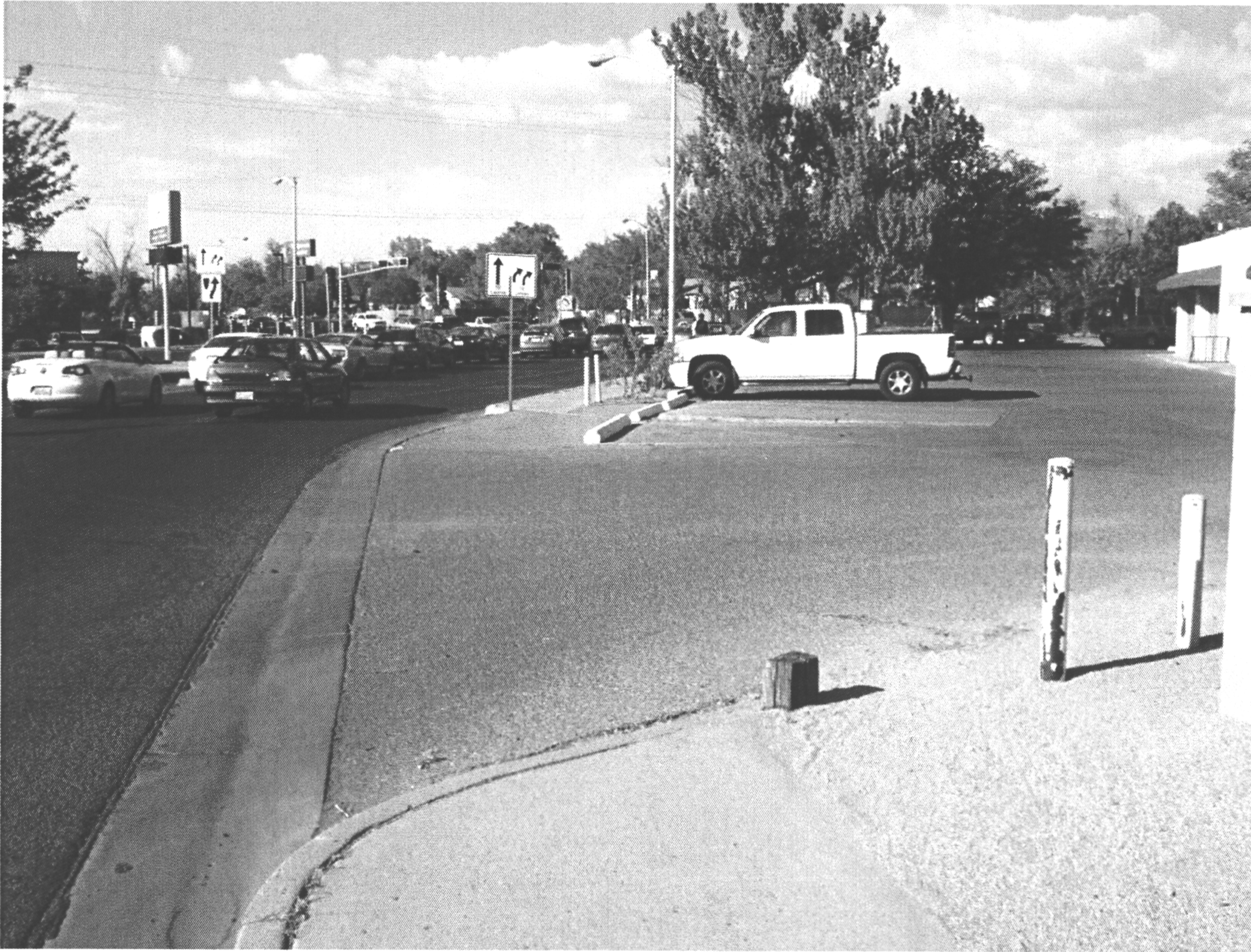
Alley intersection at Monte Vista looking north toward Lomas. Asphalt paving is flush with sidewalks at both ends.
