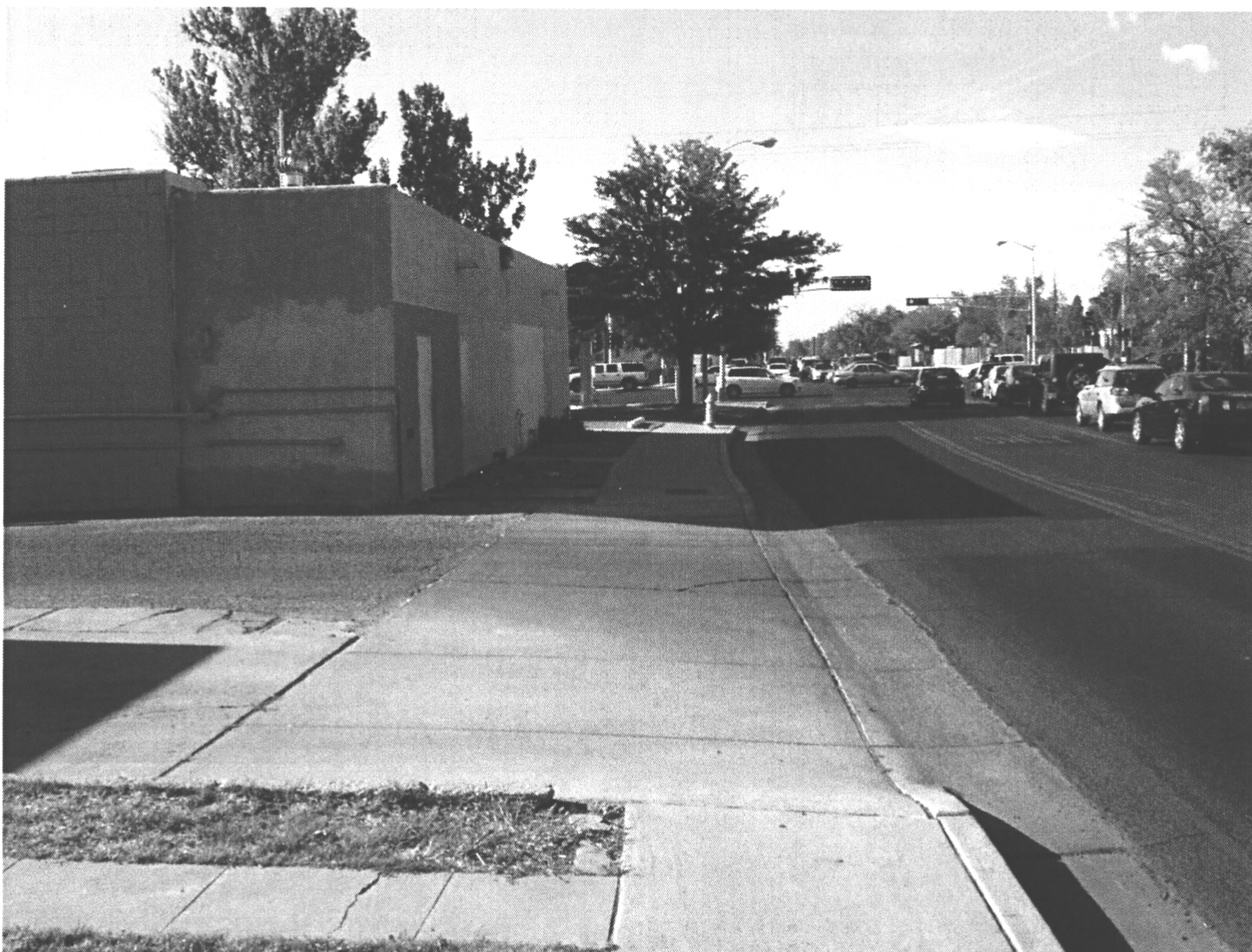
Alley entrance from Carlisle is actually a drivepad. North portion serves alley while south portion serves rental residence.
