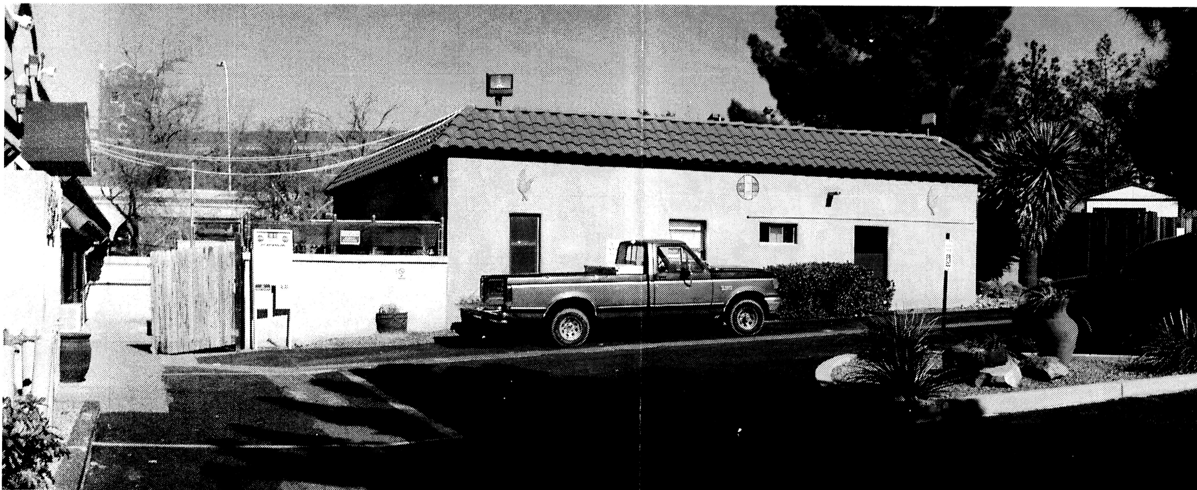
Laundry & Maintenance Building: South Elevation
