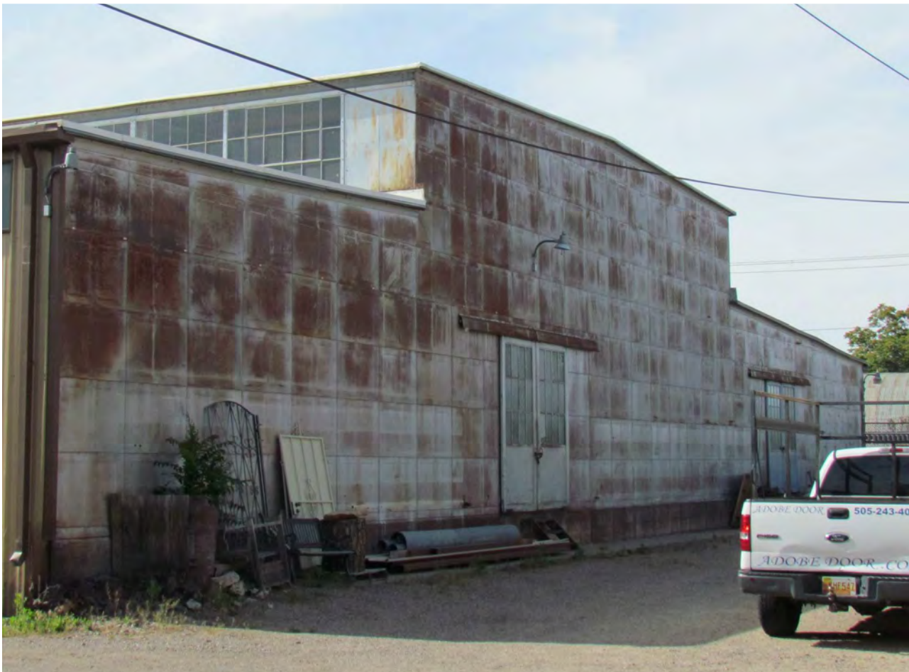
BLD "A" EXISTING WEST ENTRY LOOKING SE - EXISTING METAL PANELS TO REMAIN THROUGHOUT.
