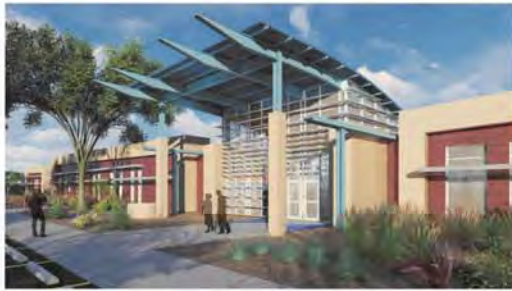
RENDERING OF SOLAR PV ARRAY OVER ENTRANCE AND EXISTING EXTERIOR
