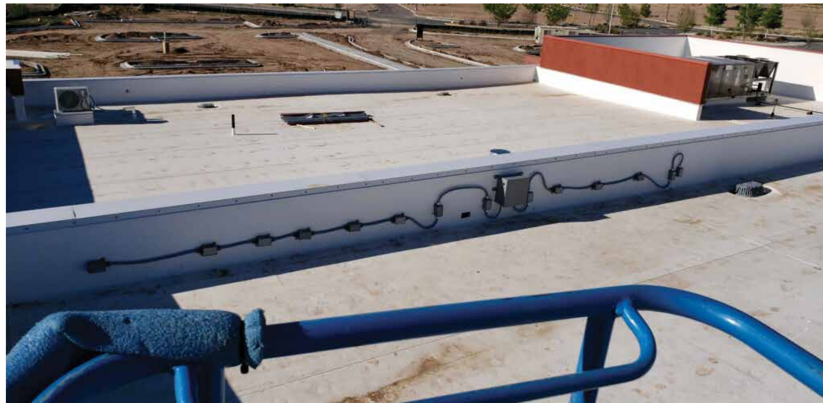
Final electrical set-up
