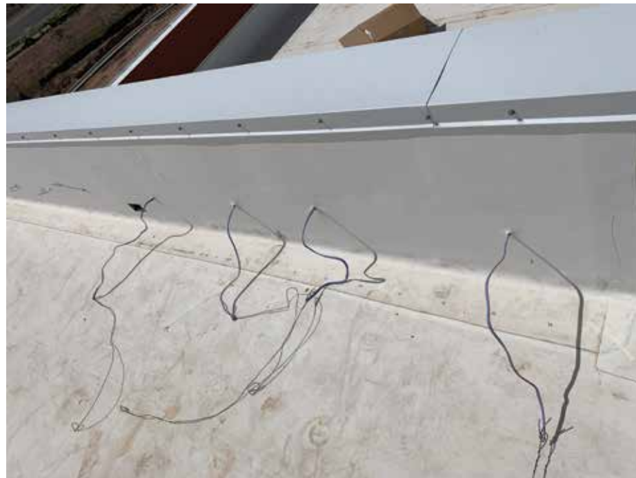
Electrical wires run through back
