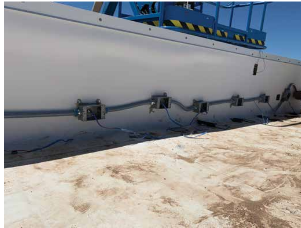
Conduit, electrical boxes, and wire set-up
