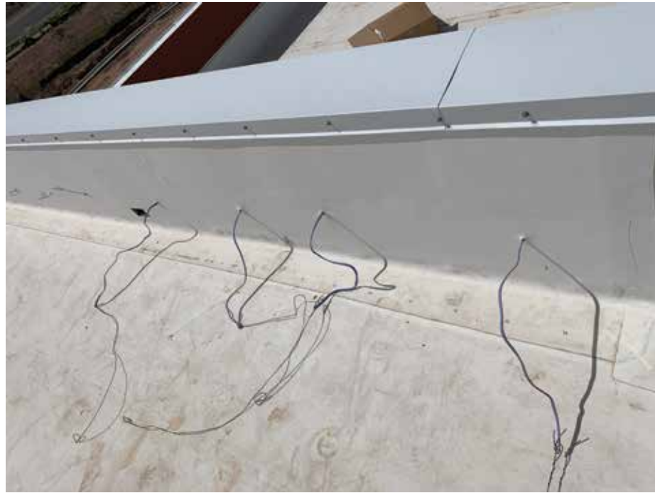
Electrical wires run through back
