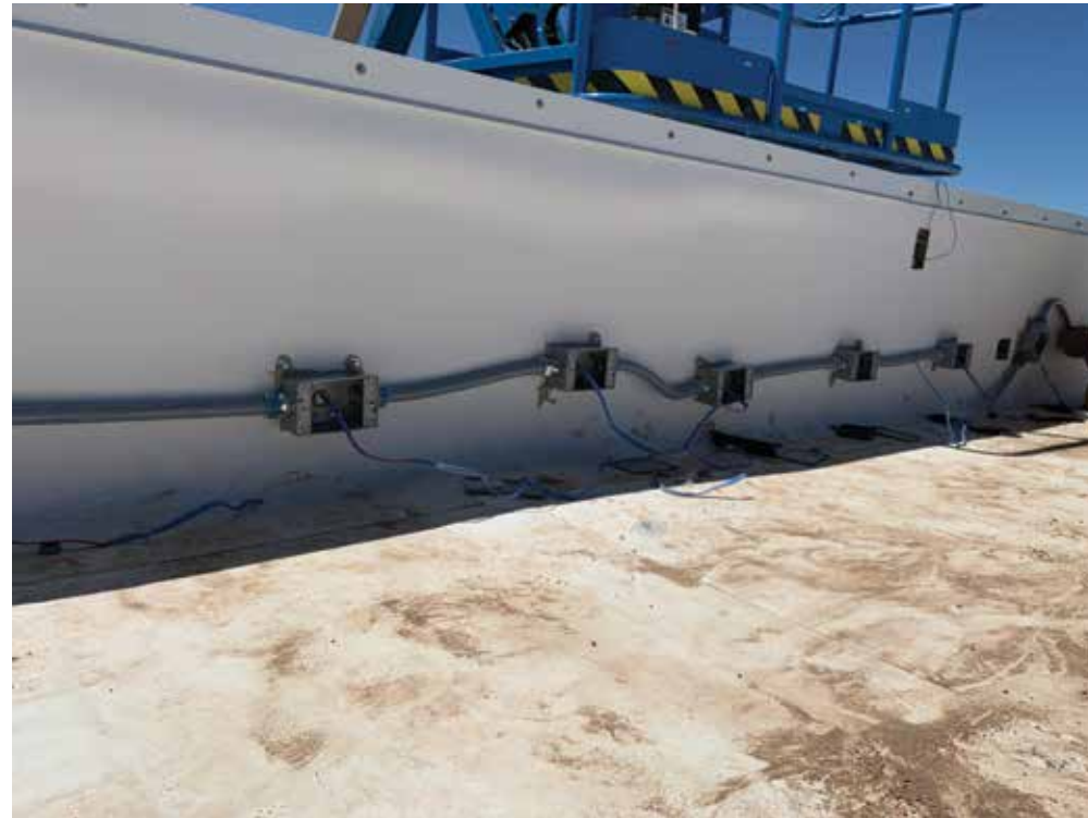
Conduit, electrical boxes, and wire set-up
