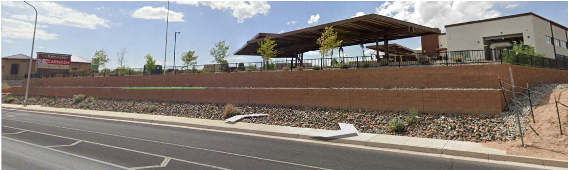
Photo 1: View to the west from Coors Blvd NW
