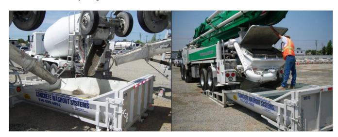
The sample spec below is intended to assist contractors, job site managers and architects with defining the concrete washout management portion of an overall Storm Water Pollution Prevention Plan (SWPPP) to meet National Pollutant Discharge Elimination System (NPDES) requirements.
