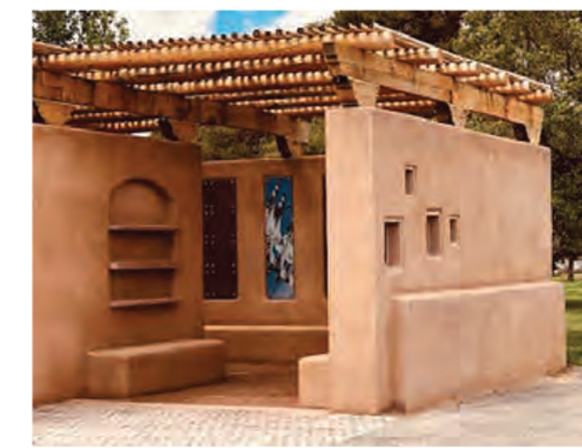
Niche Court Located Along Menaul Boulevard
