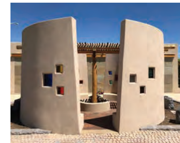
Kiva Wall Detail in Pueblo Esperanza
