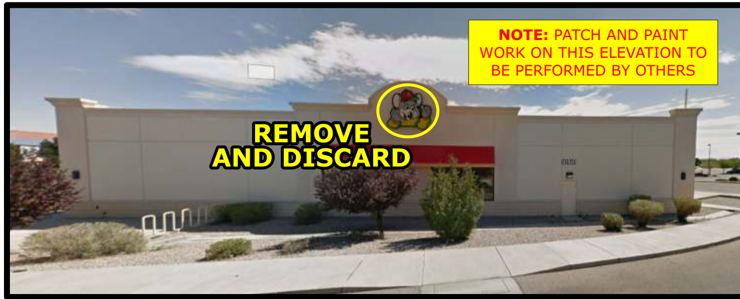
Photo Survey - Existing
