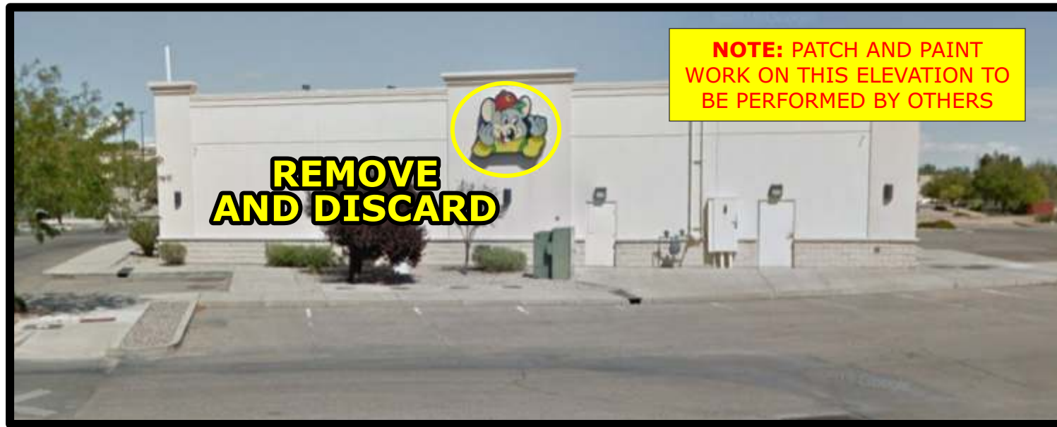
Photo Survey - Existing
