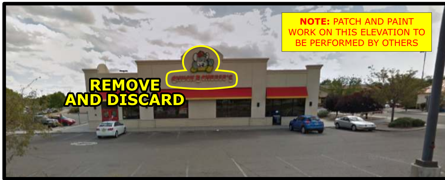
Photo Survey - Existing
