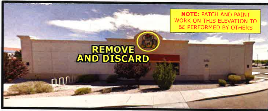
Photo Survey - Existing
