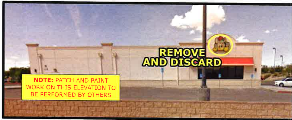
Photo Survey - Existing
