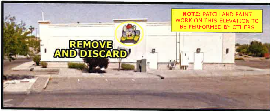
Photo Survey - Existing
