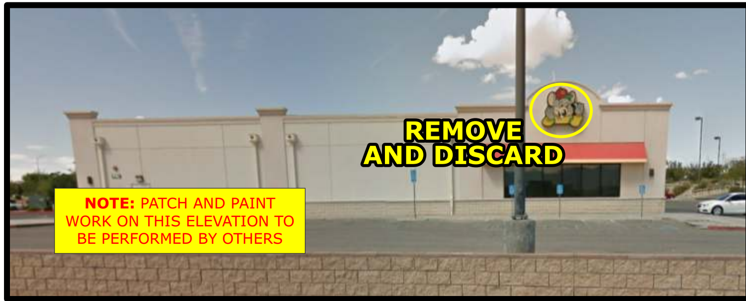
Photo Survey - Existing
