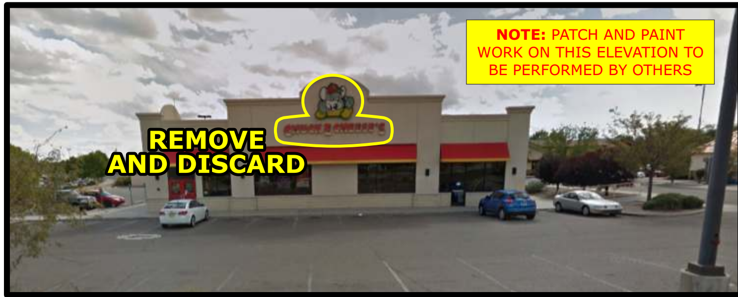
Photo Survey - Existing
