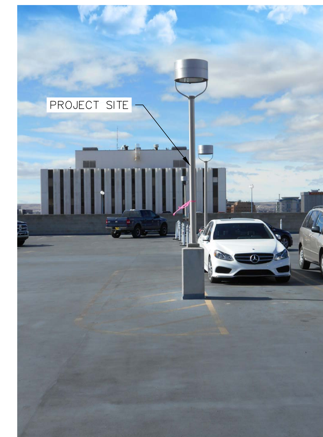
LOOKING AT PROPOSED REPLACEMENT POLE FROM EAST AT PARKING LOT:
