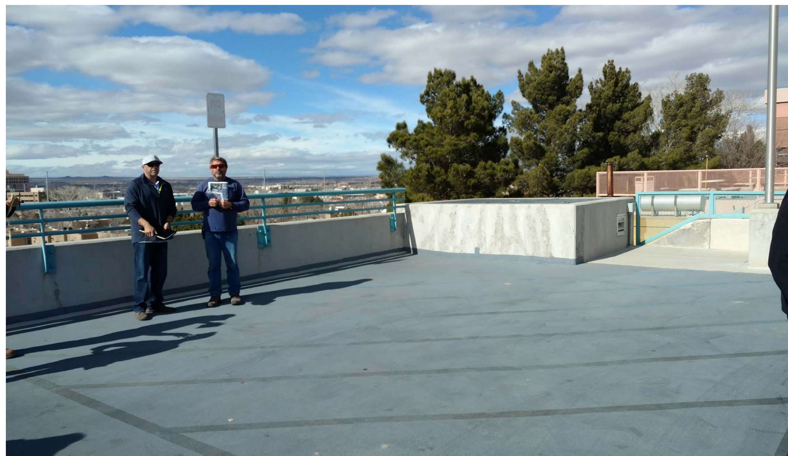
LOOKING AT PROPOSED EQUIPMENT CABINET LOCATION FROM SOUTHEAST AT PARKING LOT:
