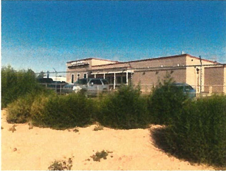
Rio Grande West Looking North
