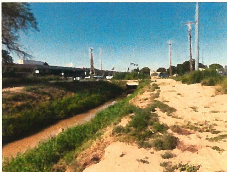
Alameda Drain Southern Reach
