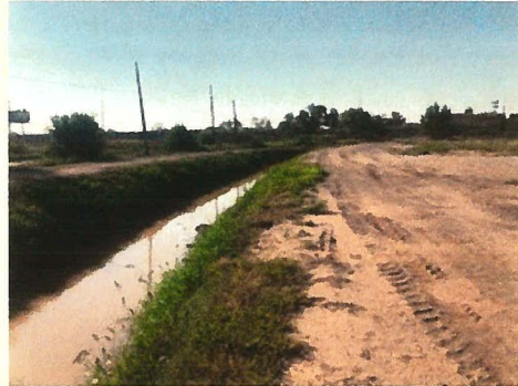
Alameda Drain Looking South
