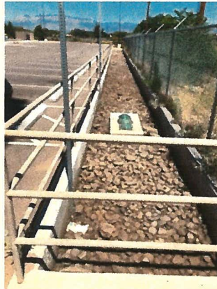
Existing Sediment Pond (South of Tract 5)
