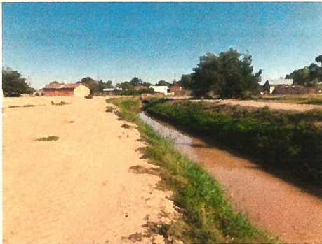
Alameda Drain Looking North
