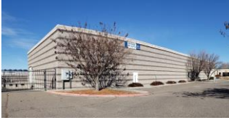
Office and Warehouse Holdings, LLC
