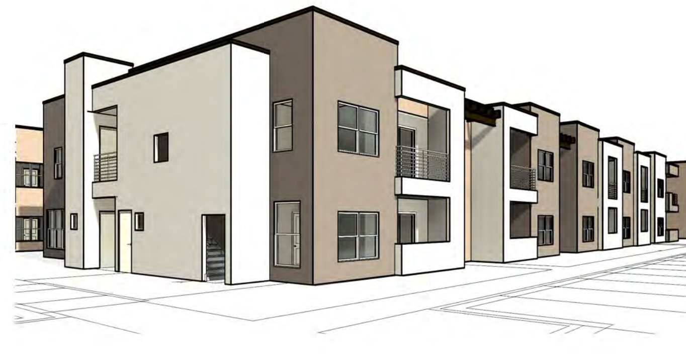
BUILDING 4 SW ELEVATION
