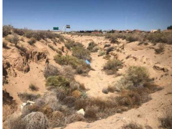
EXISTING ARROYO WITH ACCUMULATED TRASH/TUMBLE WEEDS
