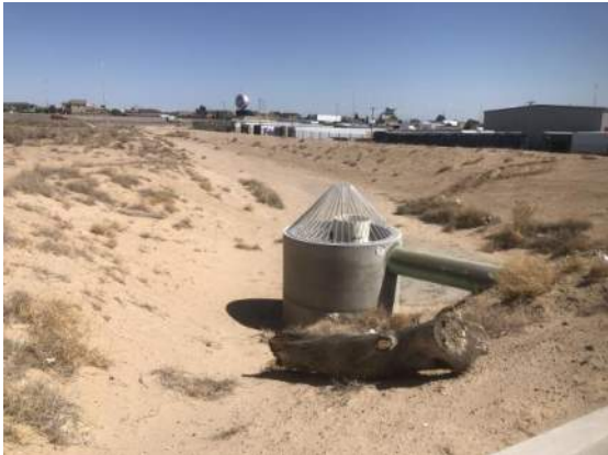
EXISTING DRAINAGE SWALE / SEDIMENT POND ALONG EAST PROPERTY LINE
