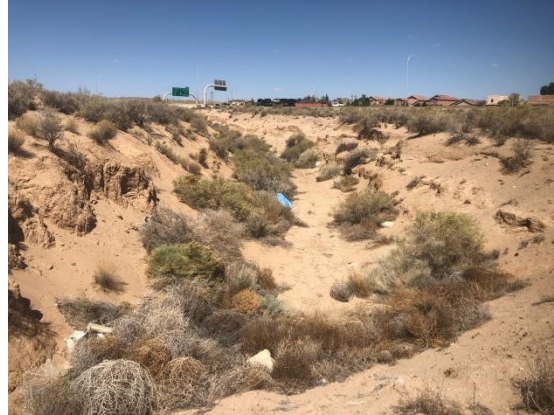
EXISTING ARROYO WITH ACCUMULATED TRASH/TUMBLE WEEDS
