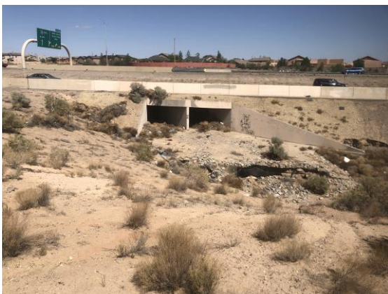
CONCRETE BOX CULVERT WITH DRAINAGE BASIN DIVERTED NORTH OF I-40
