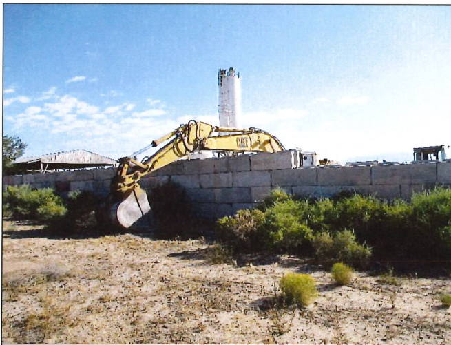
21. East adjacent property
