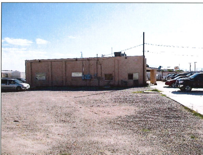
23. East adjacent property
