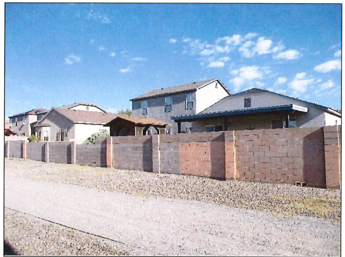
20. North adjacent property
