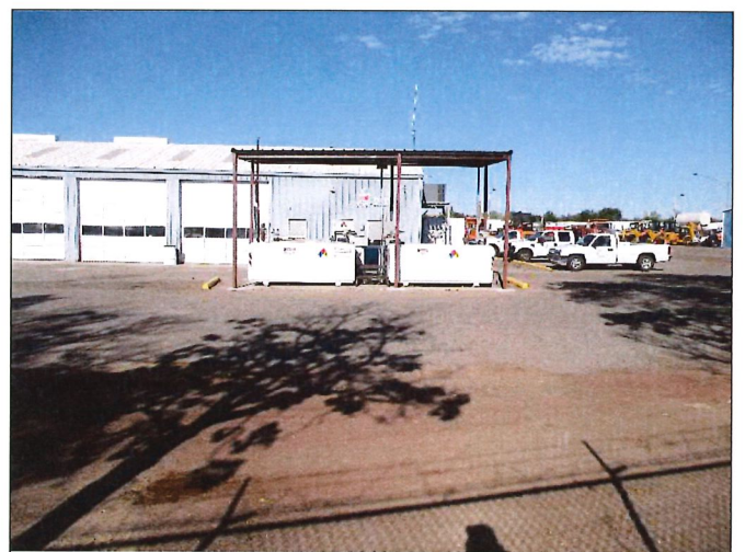
18. ASTs on west adjacent property
