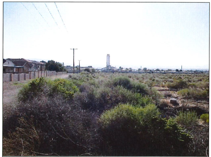
8. Northwest corner looking east
