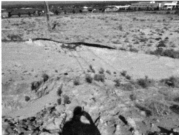
Channel flows into the property from the drainage outlet at north east corner of property.
