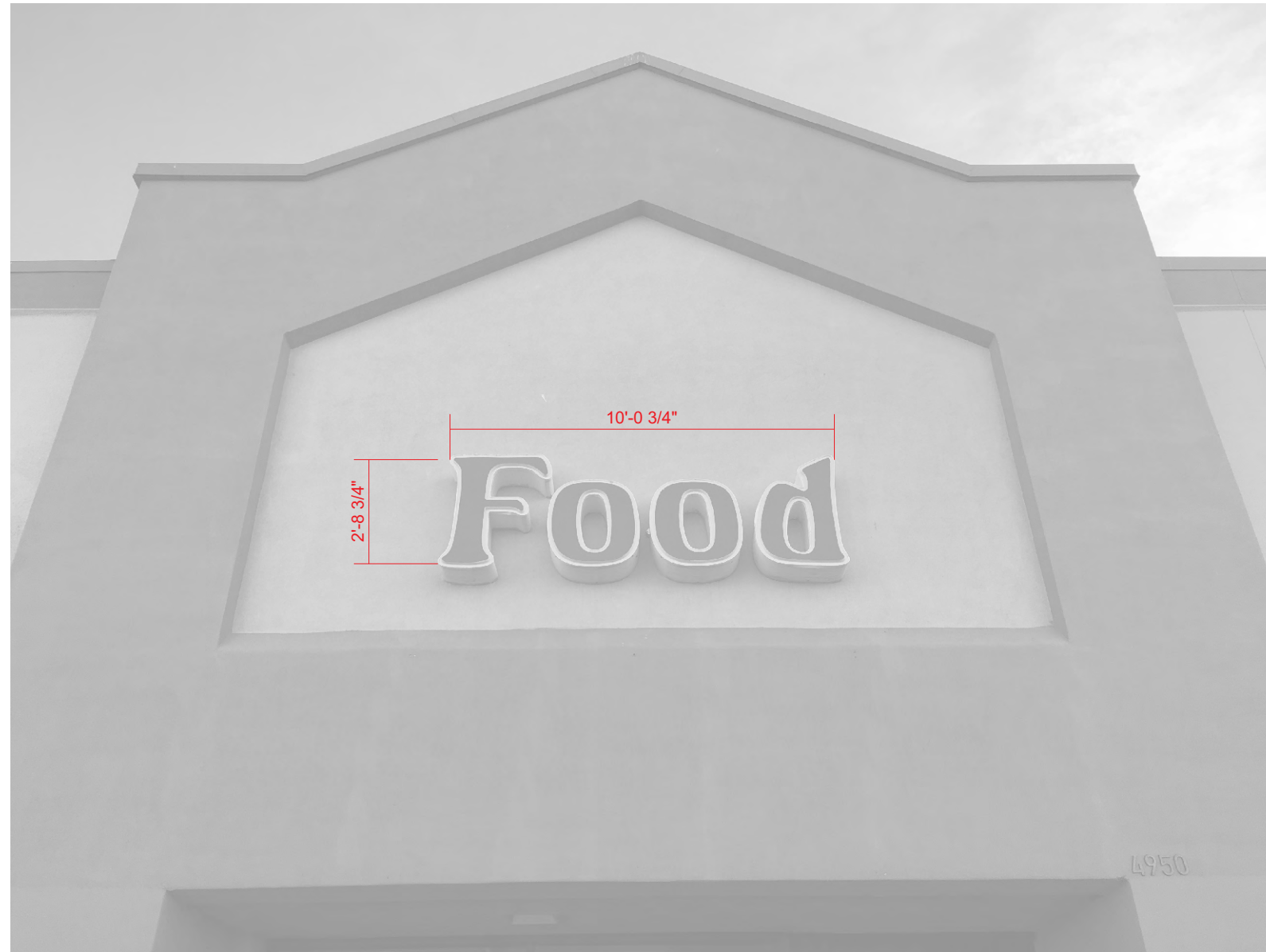
C EICL - EXISTING ILLUMINATED CHANNEL LETTERS SCALE: 1/4" = 1'
