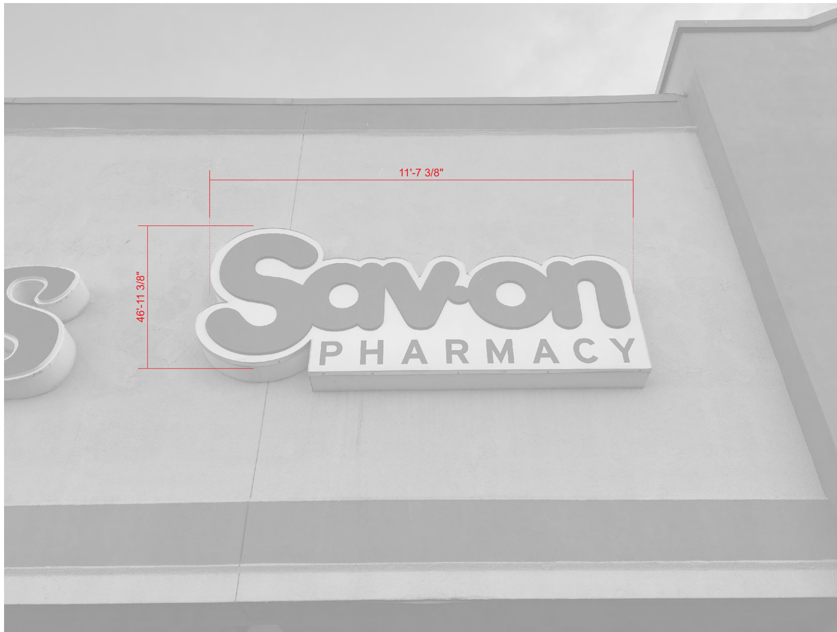
D EICL - EXISTING ILLUMINATED CHANNEL LETTERS SCALE: 3/8" = 1'
