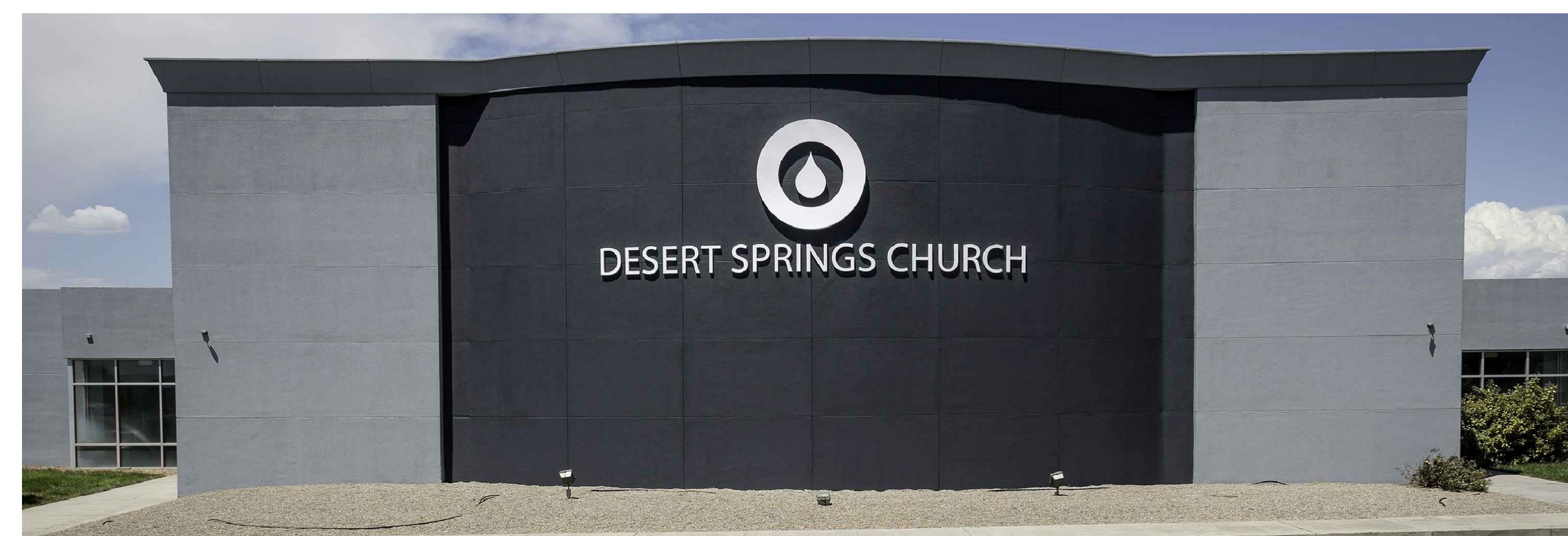
EXISTING SOUTH ELEVATION PHOTO - FOR REFERENCE
